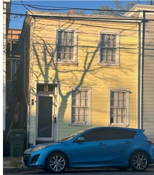
Figure 2. View of the HardiPlank siding which had been applied to the majority of the façade in September 2023. The Commission of Architectural Review did not receive any notification of this work.
