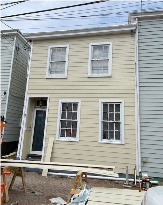
Figure 7. View of the façade of 2802 East Clay Street with new HardiPlank siding, April 2024.
