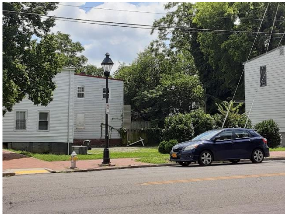
Figure 3. 421-425 North 25th Street
