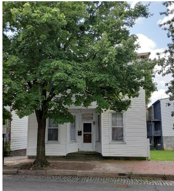
Figure 2. 2505 East Clay Street
