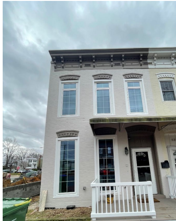
Figure 6. Front facade, 2323 Venable
