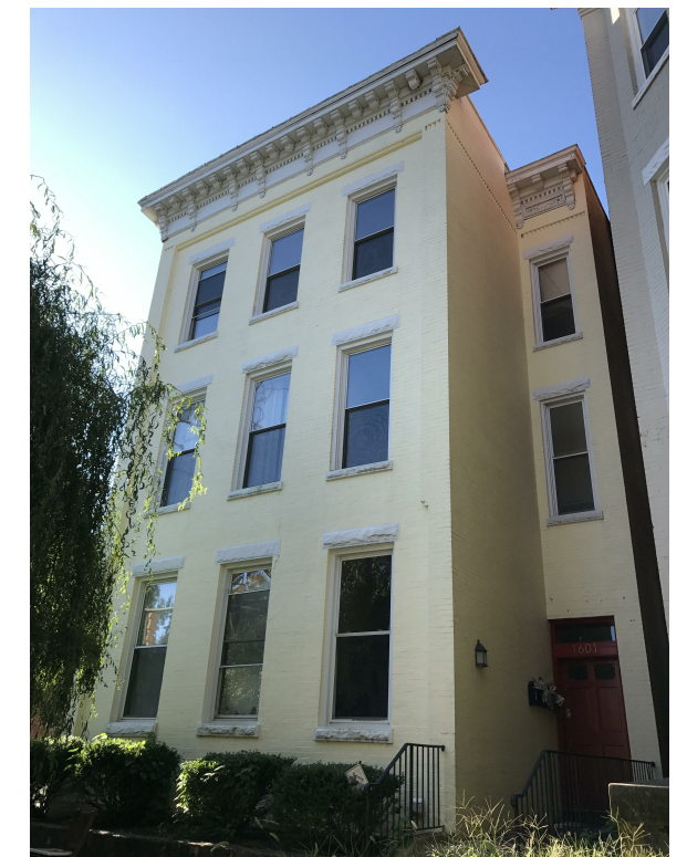
HANOVER AVE VIEW
