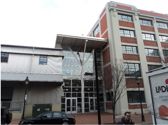
Figure 3. 101 South 15th Street, existing entrance.
