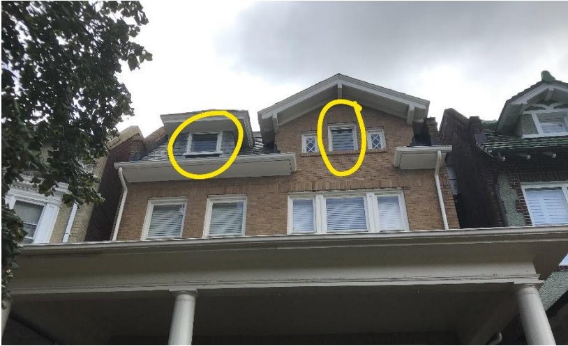
3 rd floor windows – Windows to be replaced are circled.
