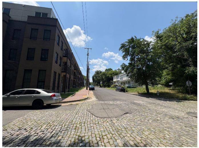
Figure 2. Looking south down Jessamine Street. Subject site on the right-hand side.
