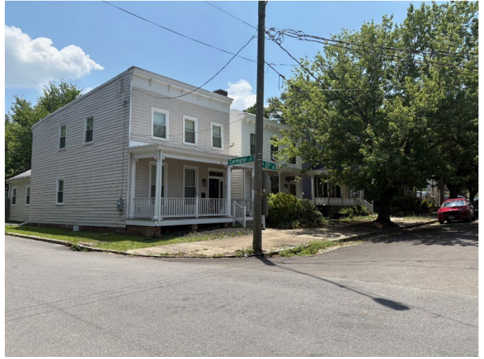
Figure 4. Residential buildings on nearby 22 nd Street, June 2025.
