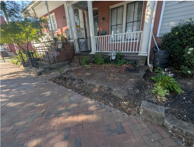
Figure 6: Current site conditions
