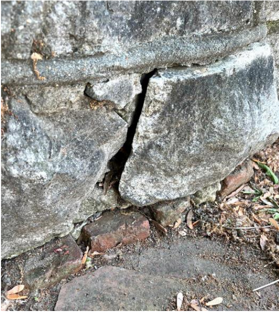
Figure 4: Site condition photograph submitted by applicant, showing an underlying layer a brick that suggests the wall was a later addition
