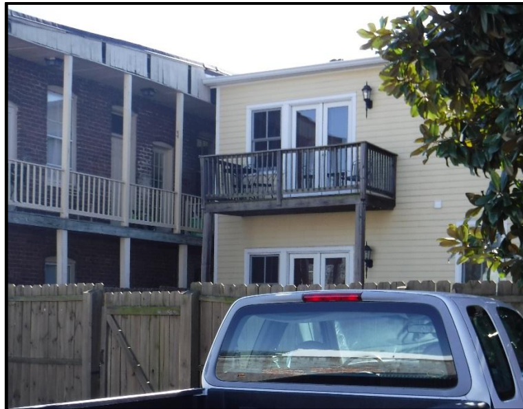
View of Rear of 318 N. 23 rd Street from Adjacent Alley (March 2018)
