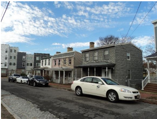
Figure 5. North side of 2000 block Cedar Street, looking northwest
