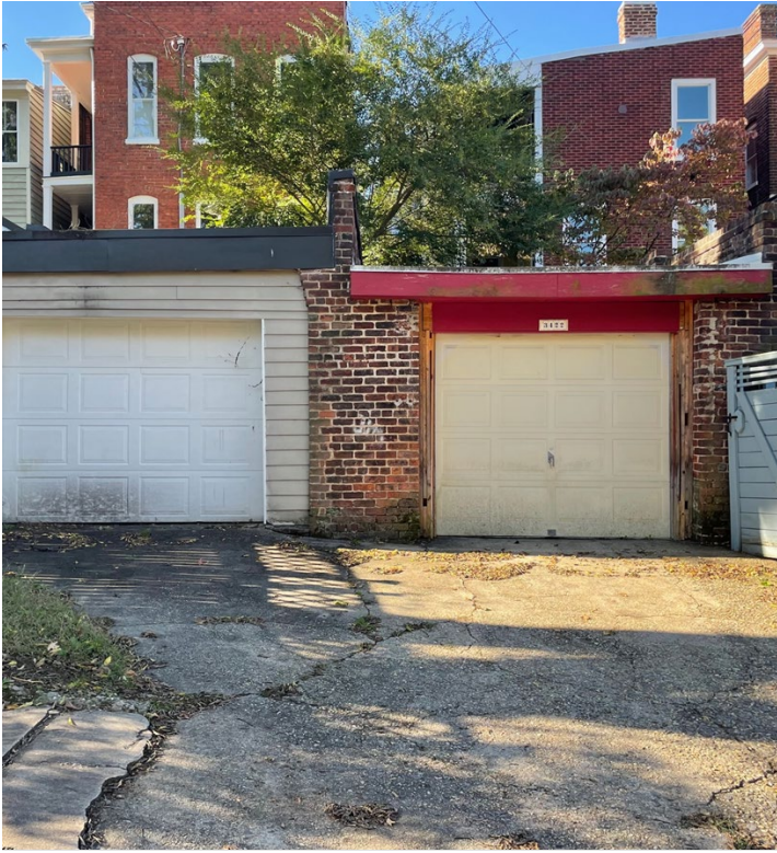
Figure 5. Garages in subject alley.
