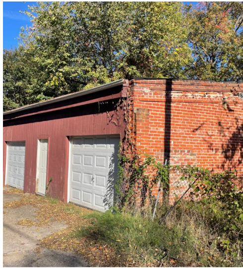
Figure 4. Out building 2710 E. Franklin
