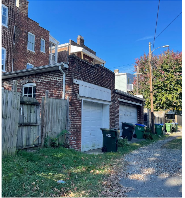
Figure 6. Garages in subject alley.
