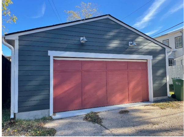
Figure 2. Out Building 108 N. 28 th Street
