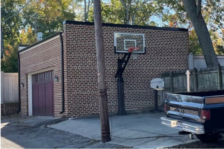
Figure 1. Out building 205 N. 28 th Street
