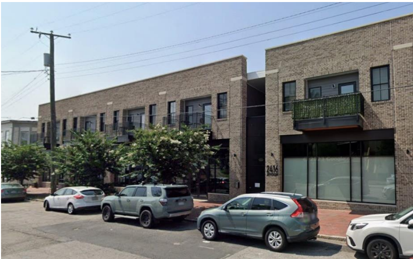
Figure 3: Balconies on 2416 Jefferson Avenue
