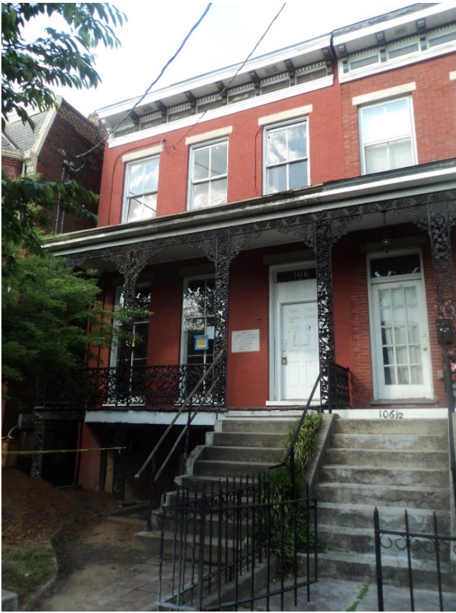
Figure 1. Facade of 106 East Clay Street.
