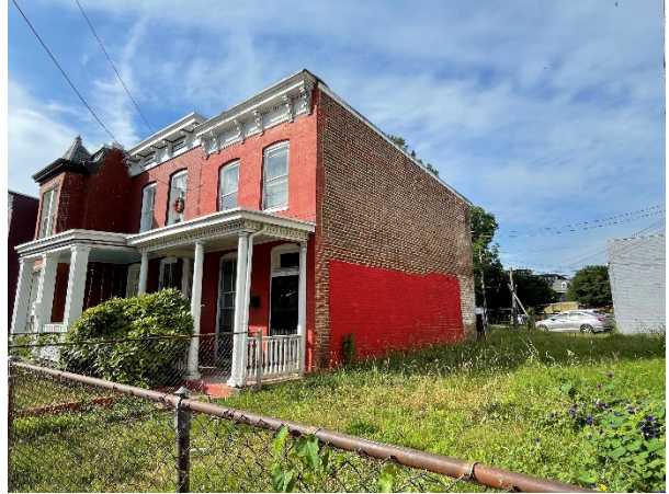
Figure 2. Side elevation of 15 W. Leigh and adjacent vacant lot.
