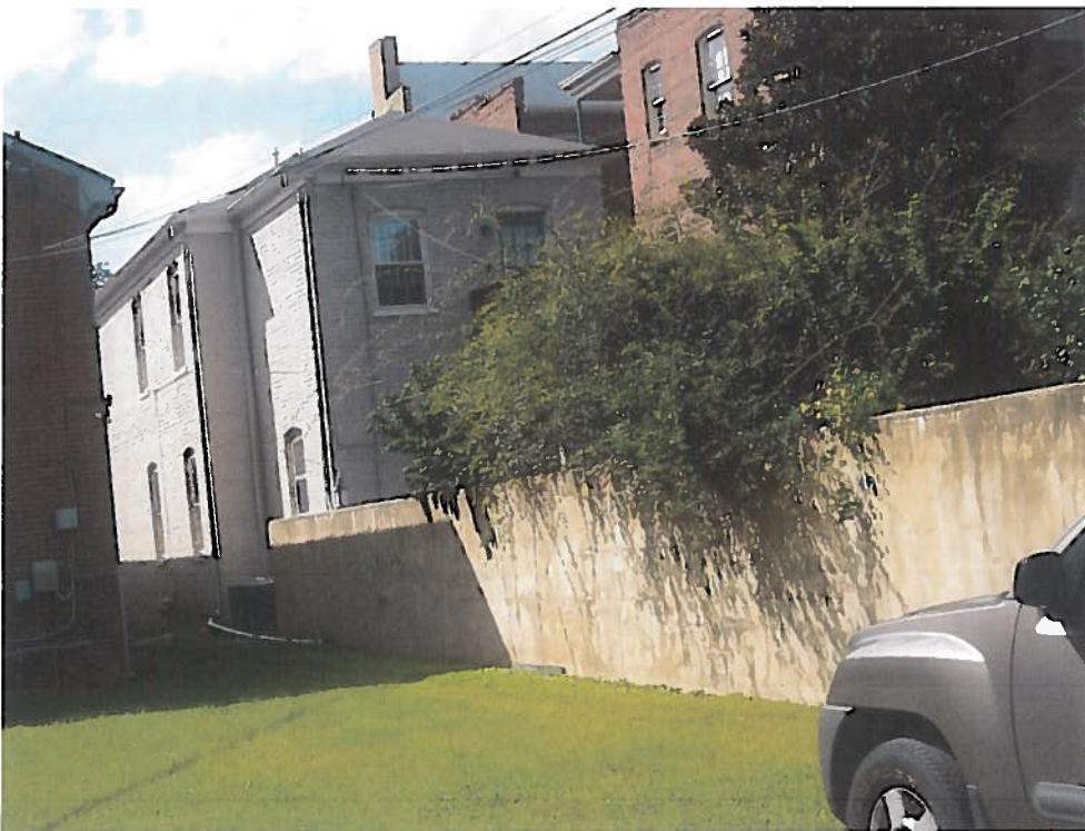
Figure 5: View of rear of house from public right of way (alley between Stuart and Kensington)
