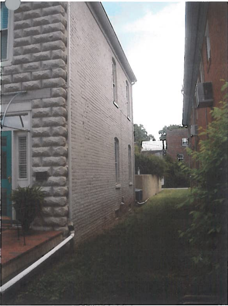
Figure 4: View of south side of building from the public right of way (sidewalk).
