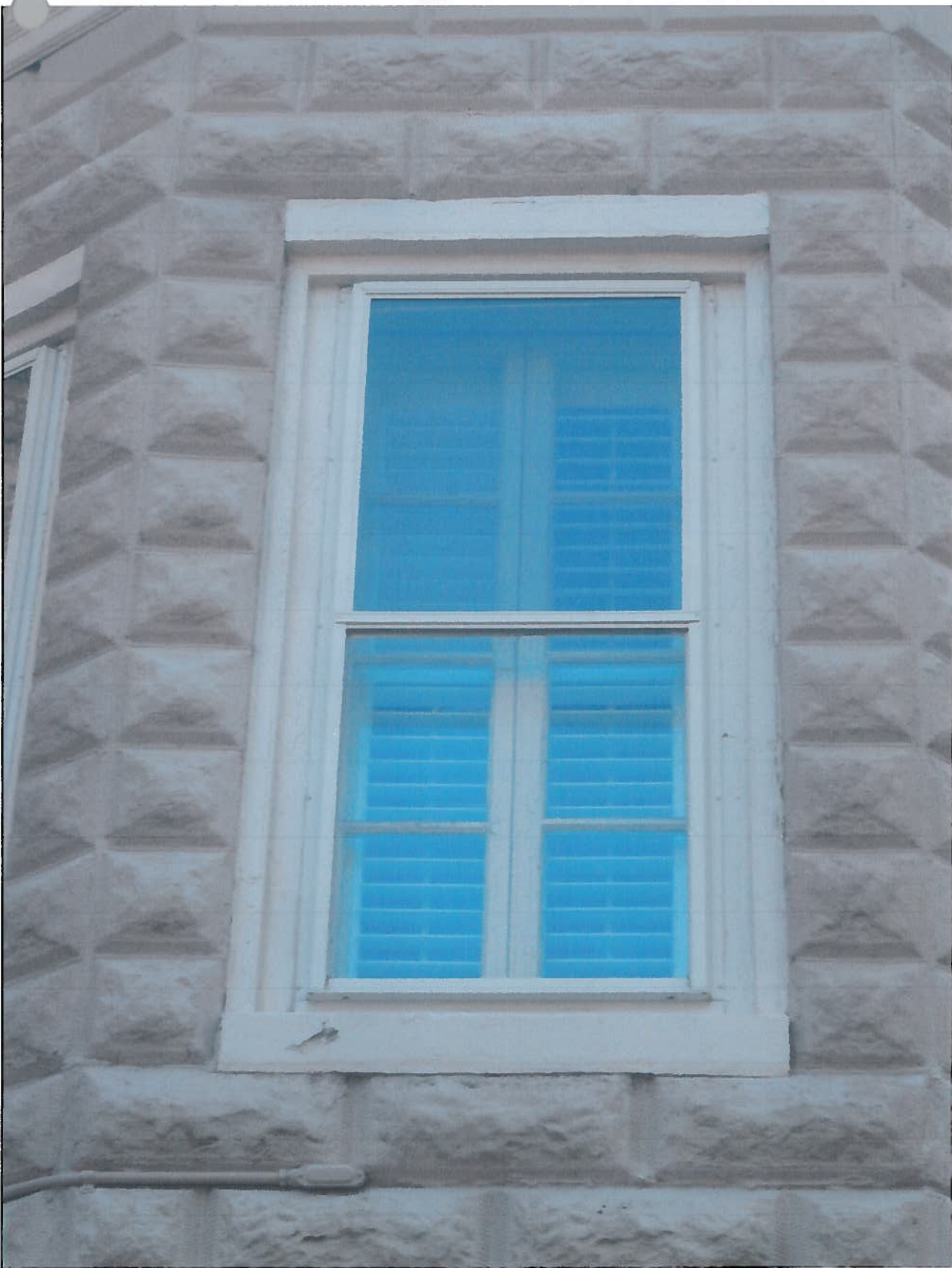
Figure 9: Existing second floor center bay window
