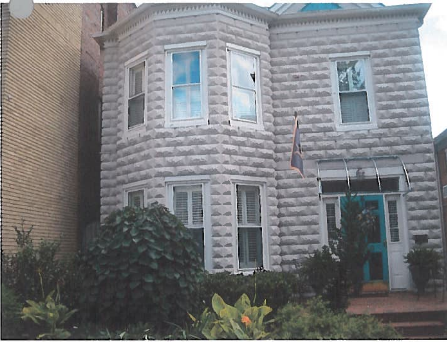
Figure 2: Front of 409 N Boulevard
