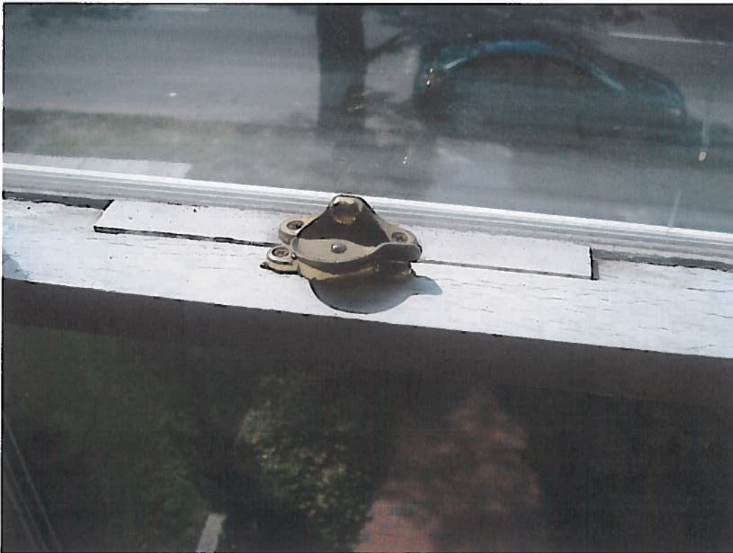
Figure 8: this is also one of the windows that needs to be shimmed to keep out the cold air in winter.
