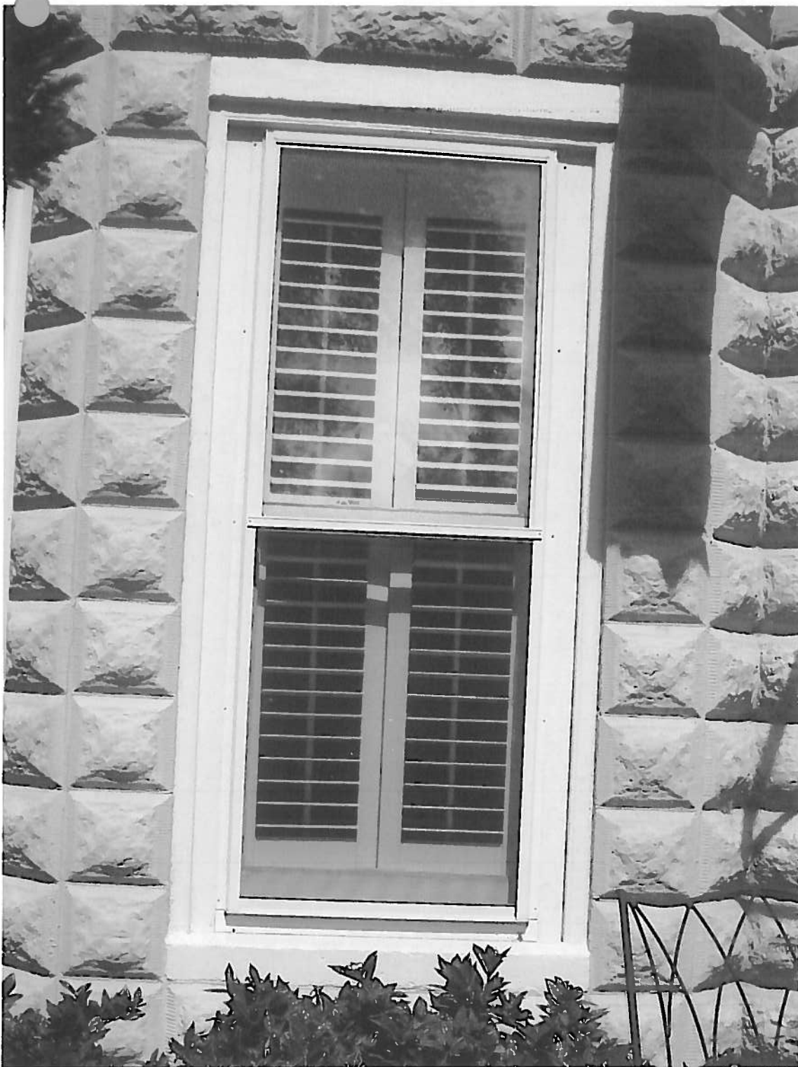
Figure 6: Close up of existing front window.
