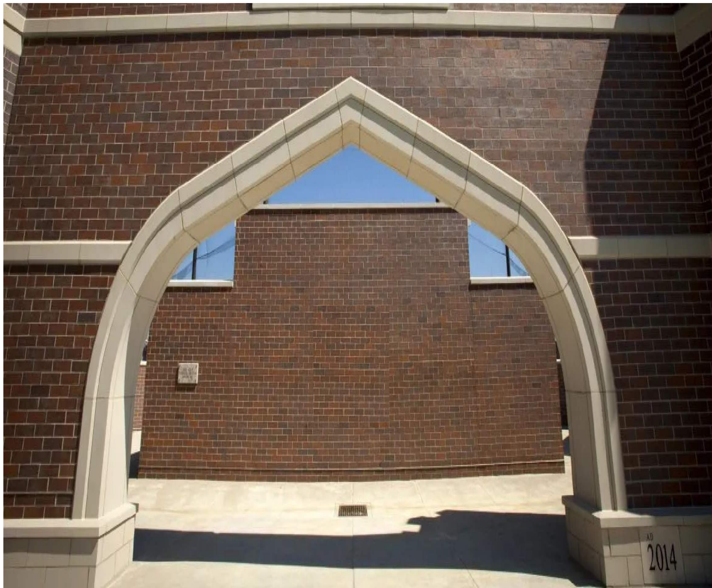
EXAMPLE: - BRICK - CAST STONE WATER TABLE - CAST STONE JAMBS, HEADERS & ARCHES - CAST STONE WALL CAPS.
