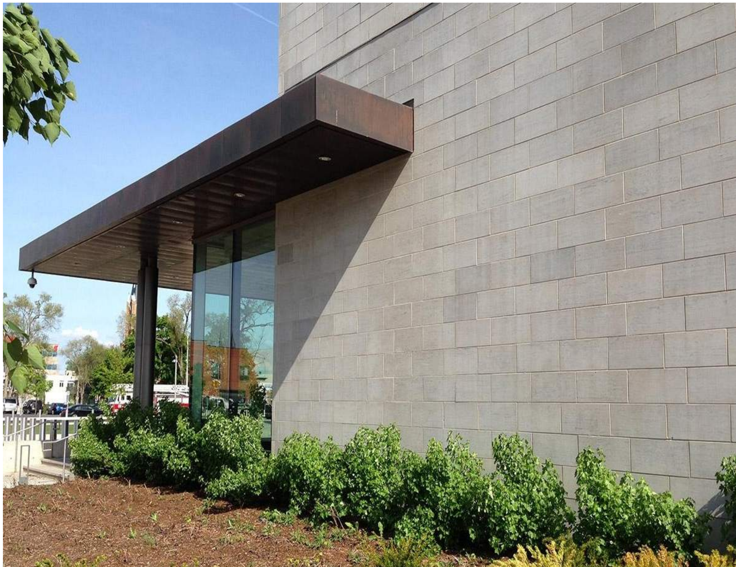
EXAMPLE: - LARGE FORMAT CAST STONE - PREFINISHED ALUMINUM COMPOSITE PANEL CANOPY SYSTEM
