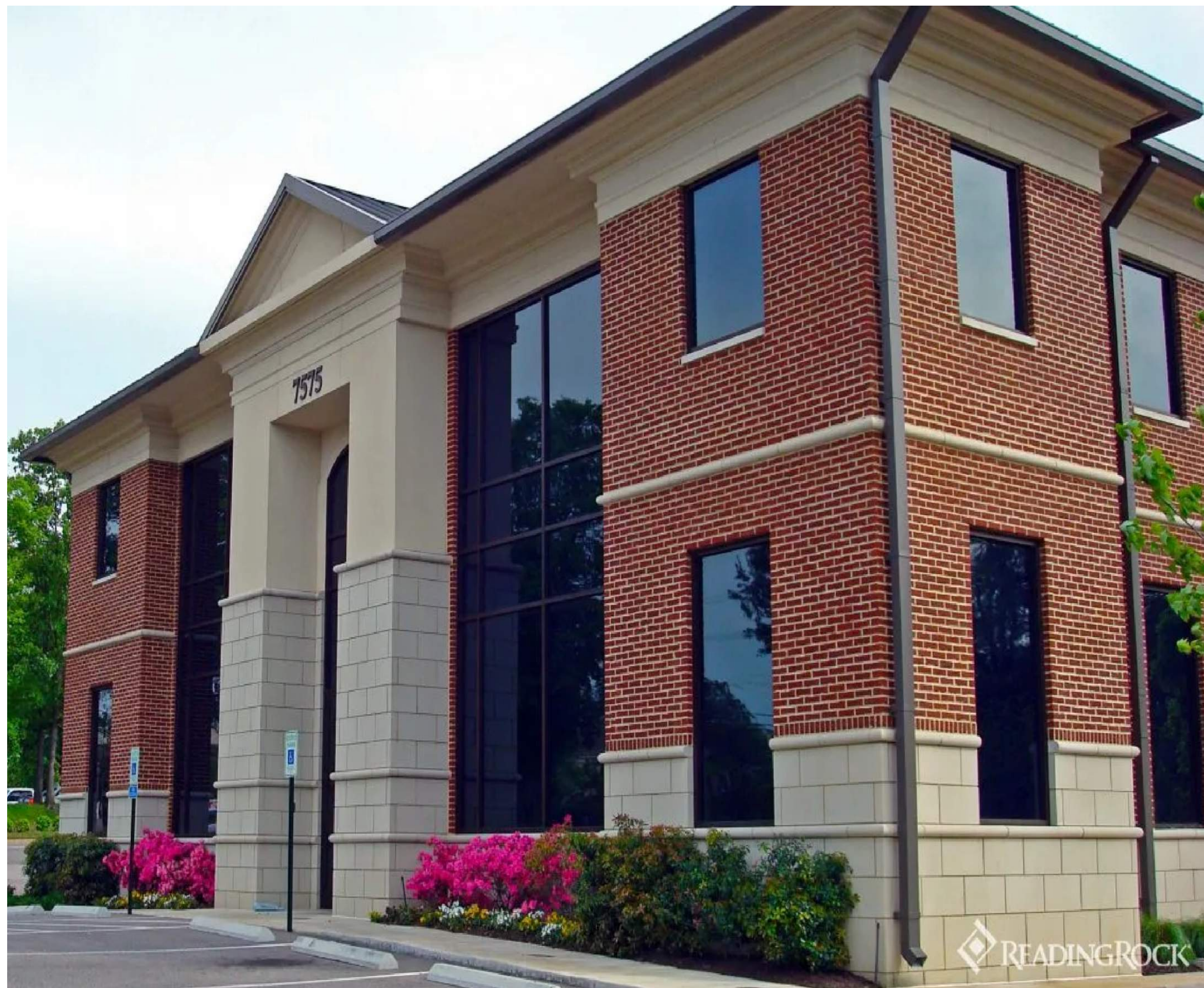
EXAMPLE: - BRICK - LARGE FORMAT CAST STONE - CAST STONE WATER TABLE & CORNICE
