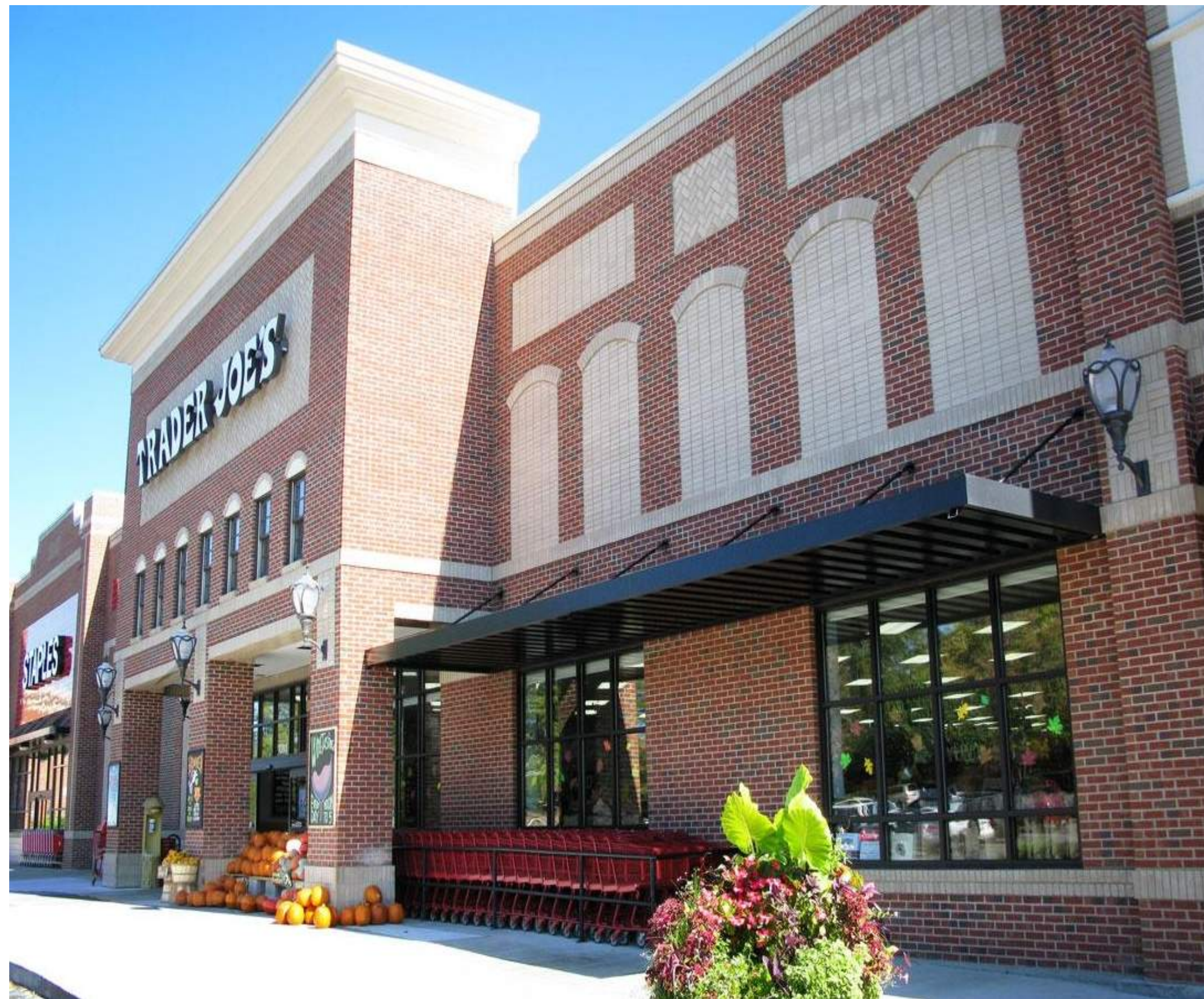
EXAMPLE: - BRICK - PREFINISHED ALUMINUM CANOPY SYSTEM
