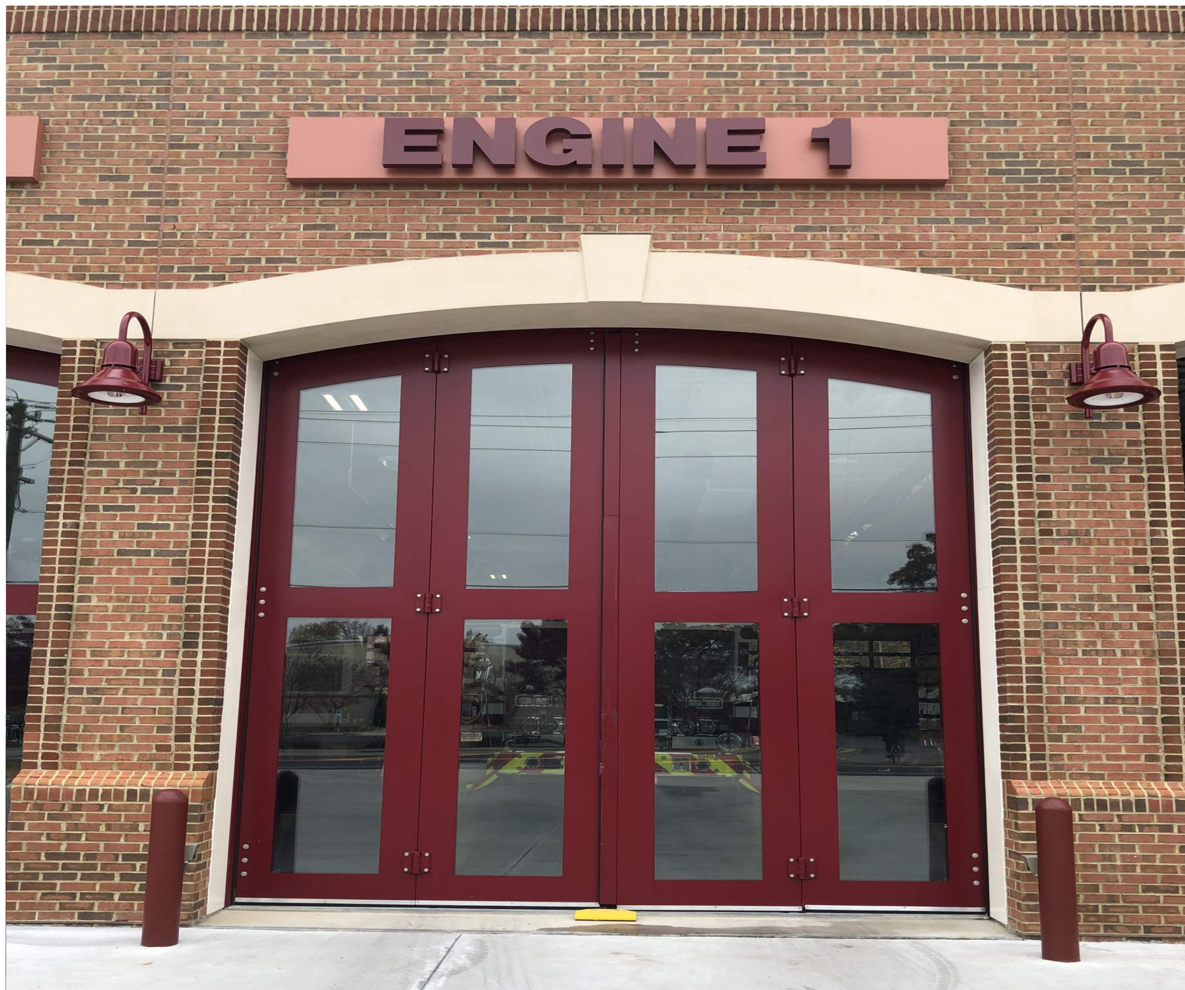
EXAMPLE: - CAST STONE HEADER - PREFINISHED APPRATUS BAY DOOR SYSTEM - PREFINISHED ALUMINUM DIMENSIONAL BACK-LIT SIGNAGE SYSTEM
