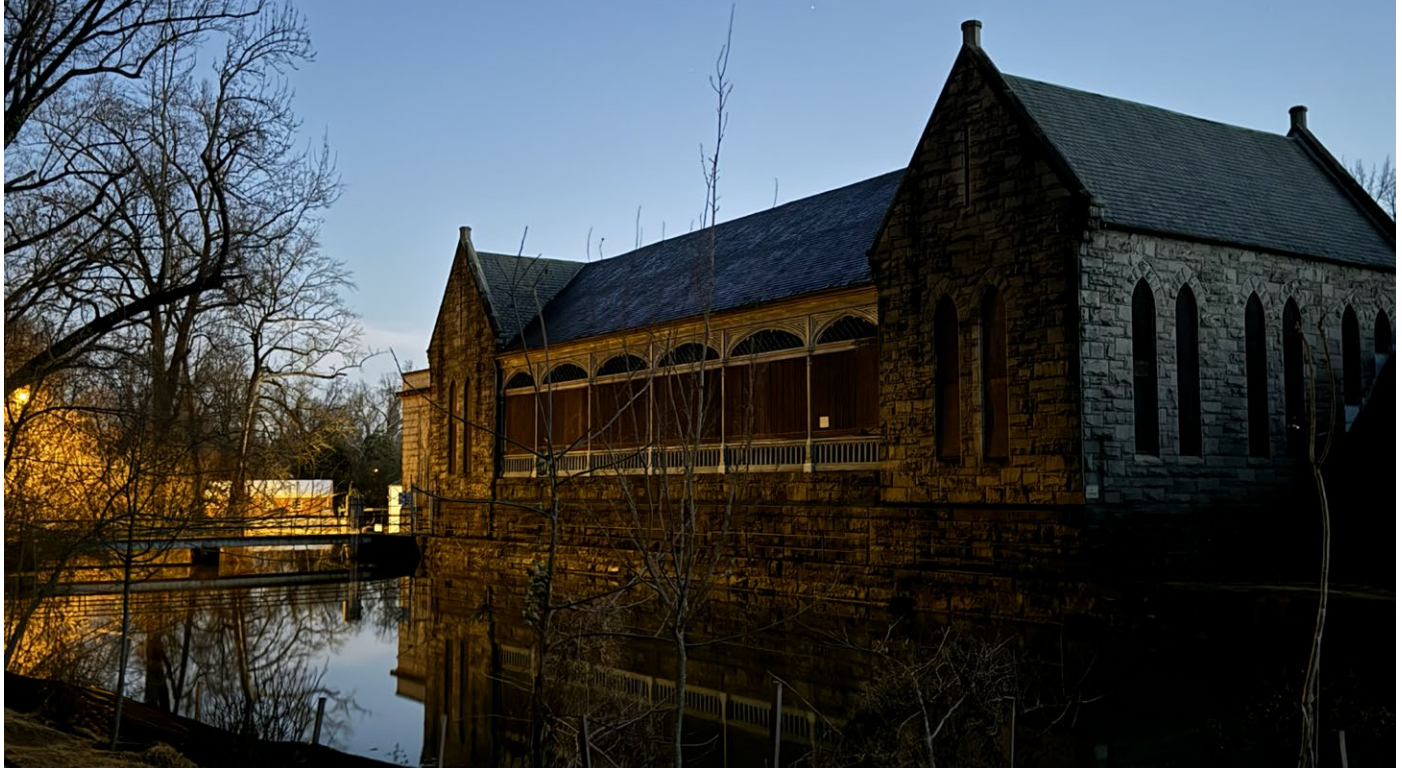
The historic pump house at Pump House Park along the Kanawha Canal
