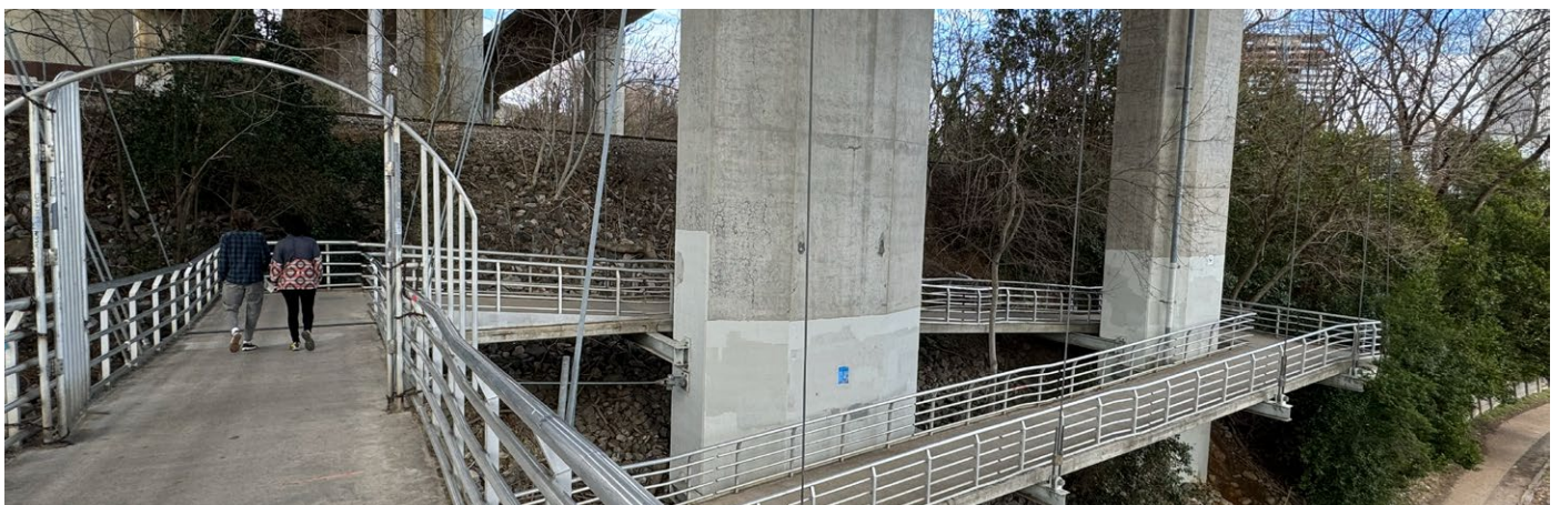
Pedestrians walk on the pedestrian bridge from Belle Isle Park
