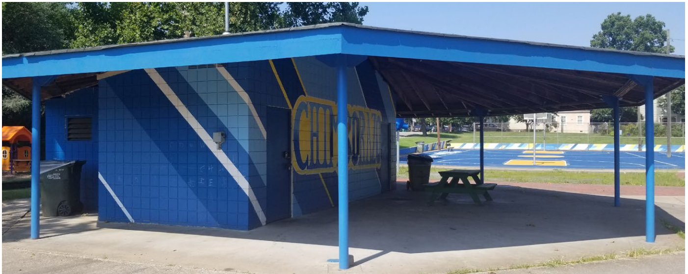
Restroom building (locked at the time of this photo) and basketball courts at Chimborazo Playground
