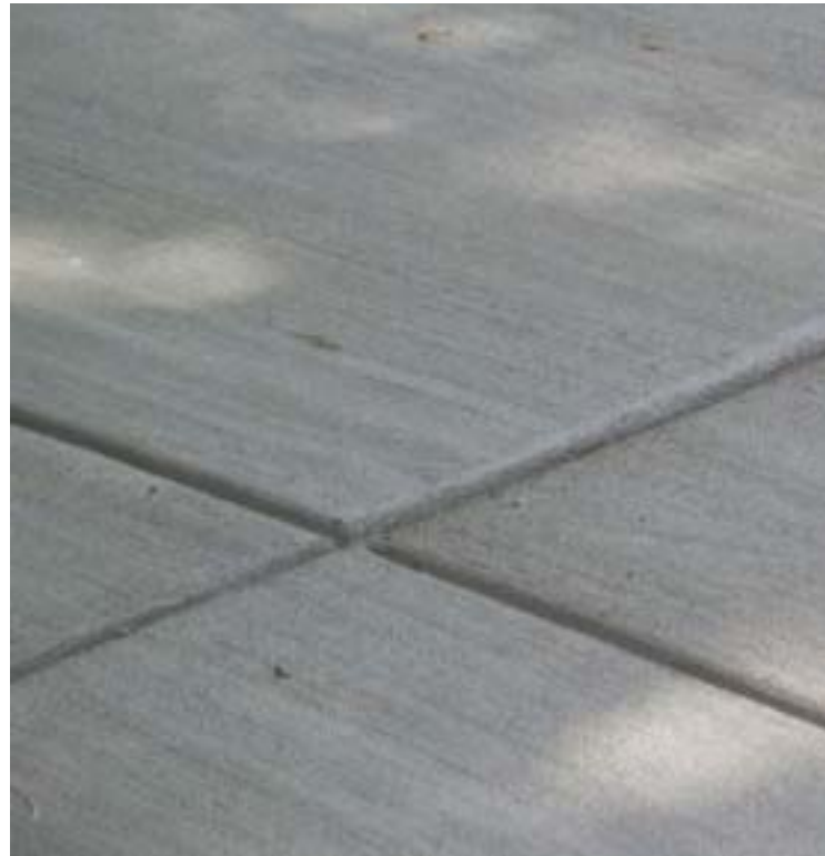
BRUSHED CONCRETE: EXISTING SIDEWALK, REPAIRED AS NEEDED, MARKS THE PATH FOR PEDESTRIANS. CONCRETE CLEARLY DEFINES DRIVEWAY ENTRANCES WHERE IT CROSSES THE BRICK PAVING.
