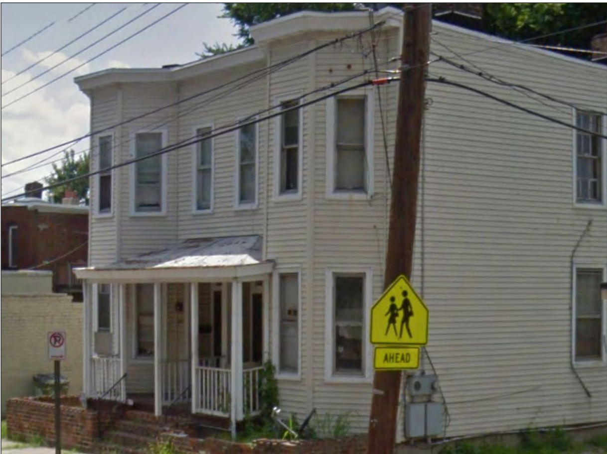
Prior to work performed - Google Streetview July 2014
