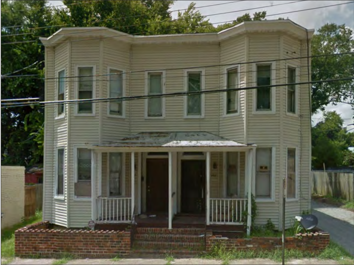
Prior to work performed - Google Streetview July 2014
