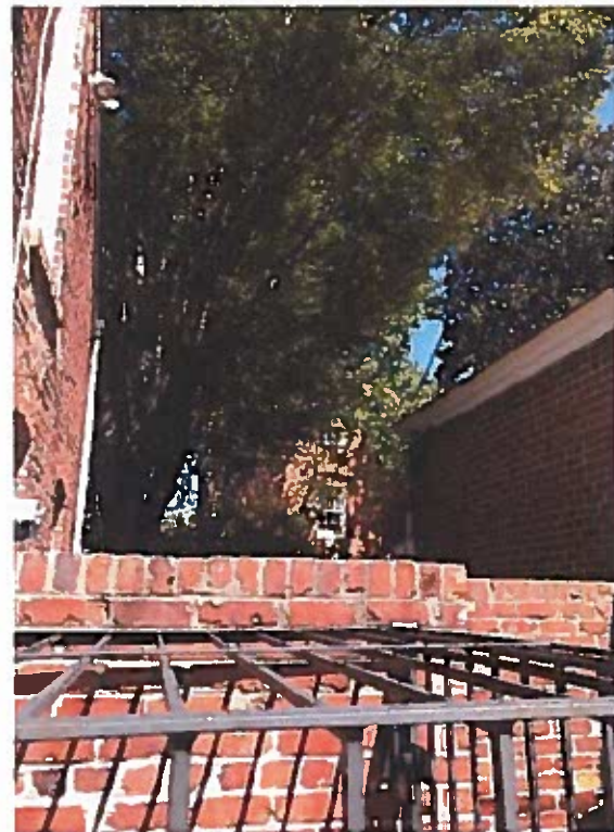
VIEW OF REAR ELEVATION FROM ALLEY
