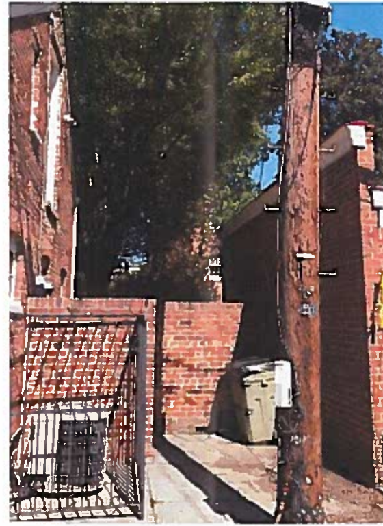
VIEW OF REAR ELEVATION FROM ALLEY
