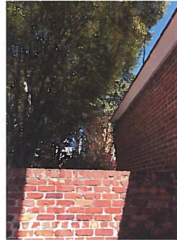
VIEW OF REAR ELEVATION FROM ALLEY
