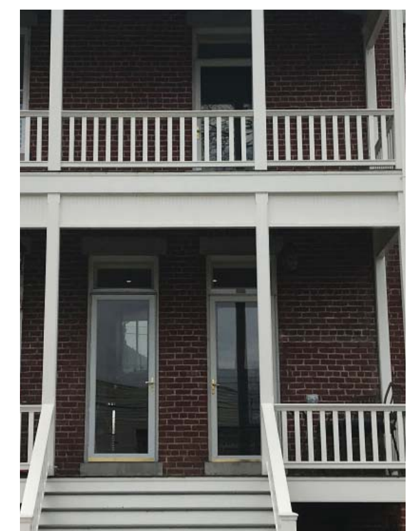
EXISTING REAR DOORS
