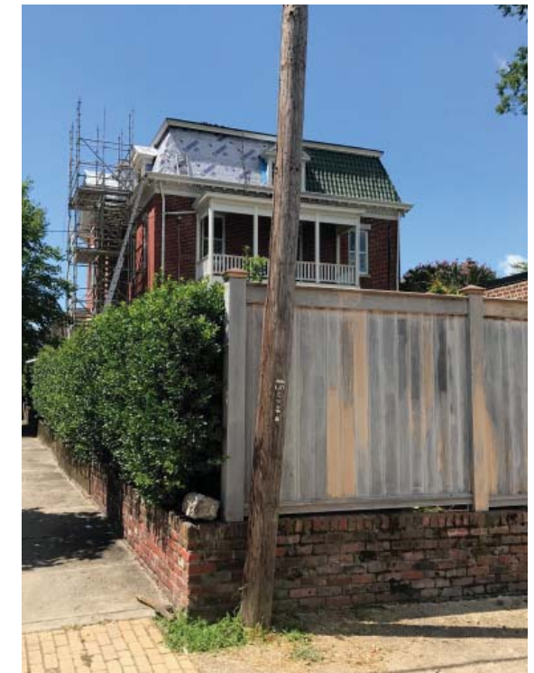
VIEW OF REAR ELEVATION FROM ALLEY
