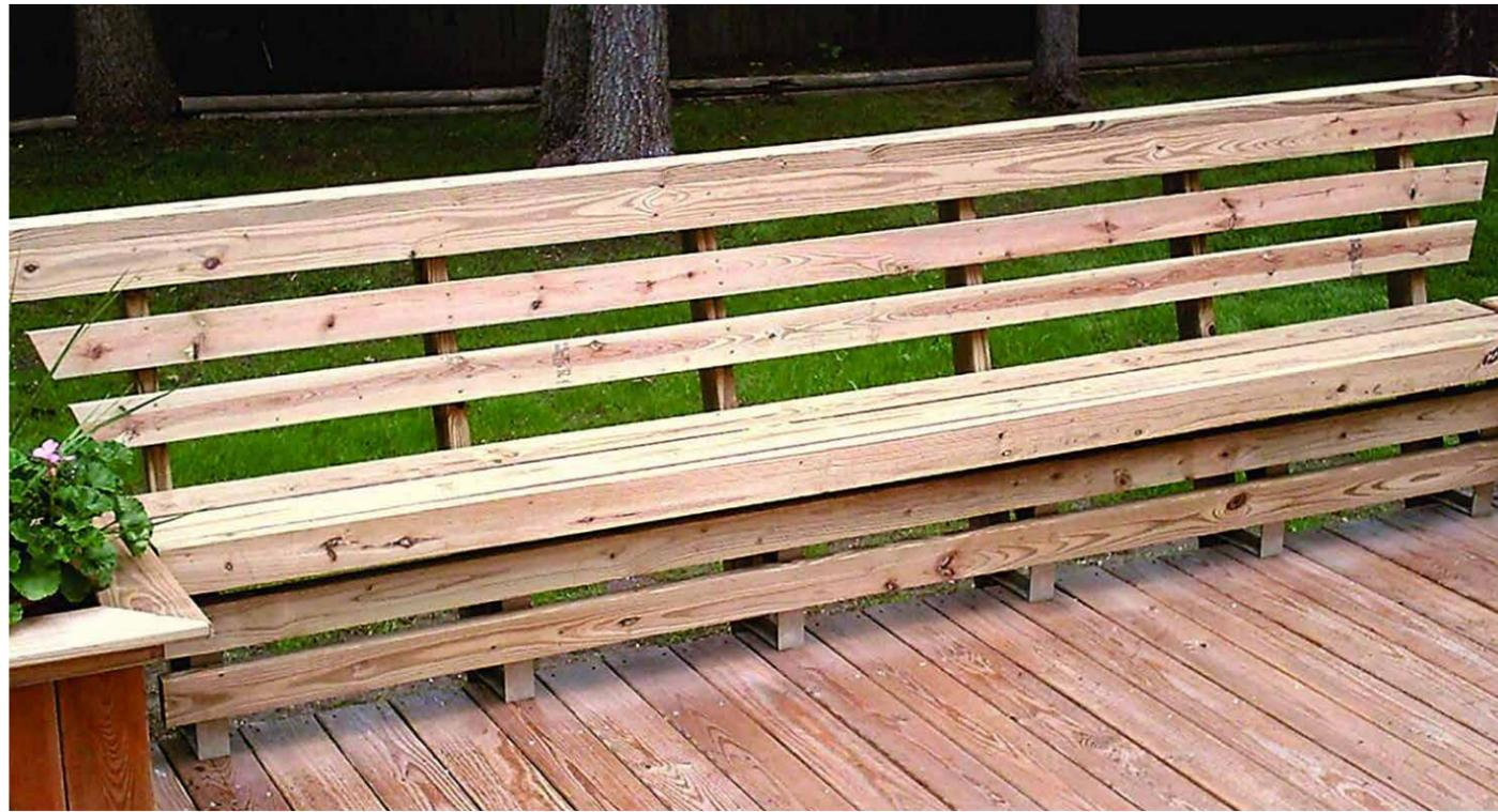
DECK BENCH SEATING - KEEP OPEN SLATS FOR VISIBILITY THROUGH BENCHES FOR SAFETY - PROVIDE BACKS FOR COMFORT AND TO ENCOURAGE USE
