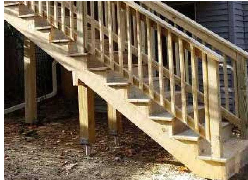
WOODEN STAIR AND RAILING - UPGRADE EXISTING RAILINGS AS NEEDED TO MEET BUILDING CODE FOR GUARDRAILS
