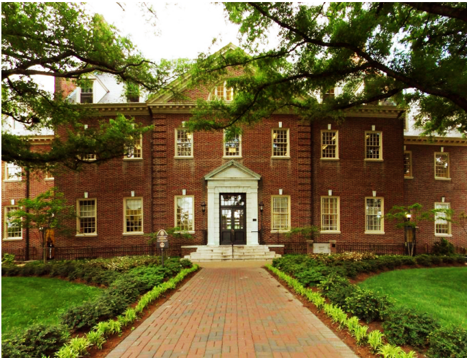
View of Bacot Hall Front Door
