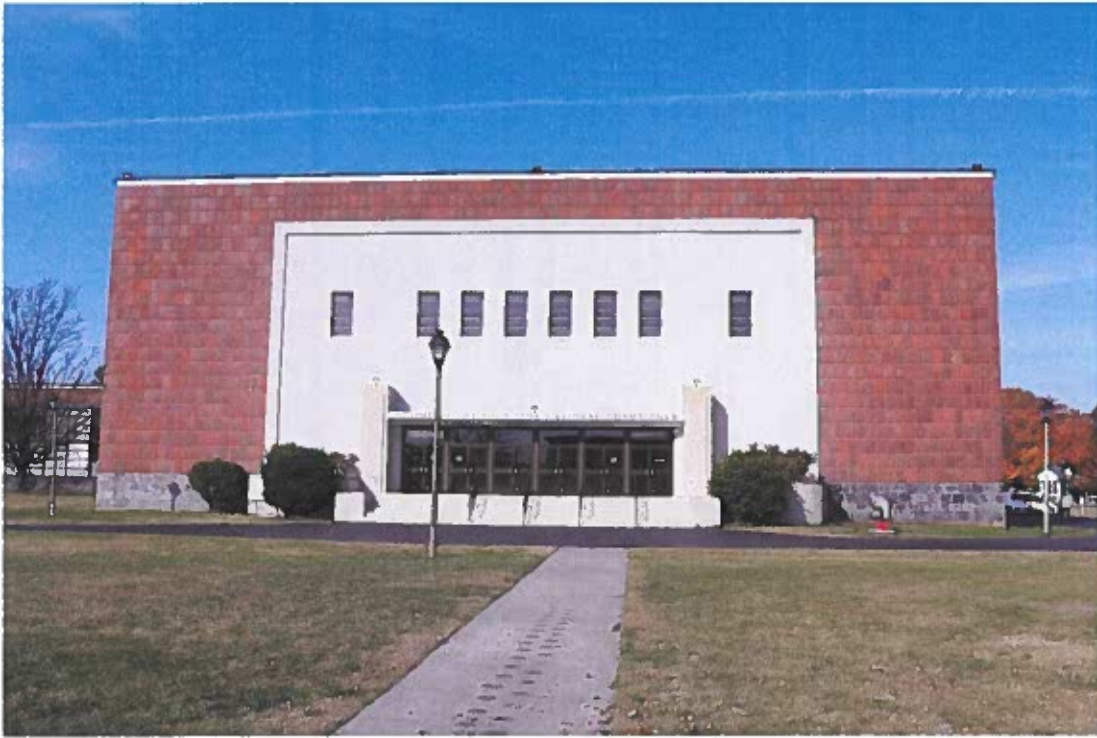
Photo 1. Southeast elevation of field house/gymnasium, looking northwest, Belgian Building, 11/17/21
