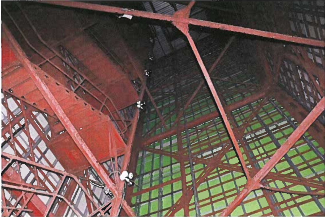
Photo 19. Upward view of bell tower structure from base, Belgian Building, 11/17/21
