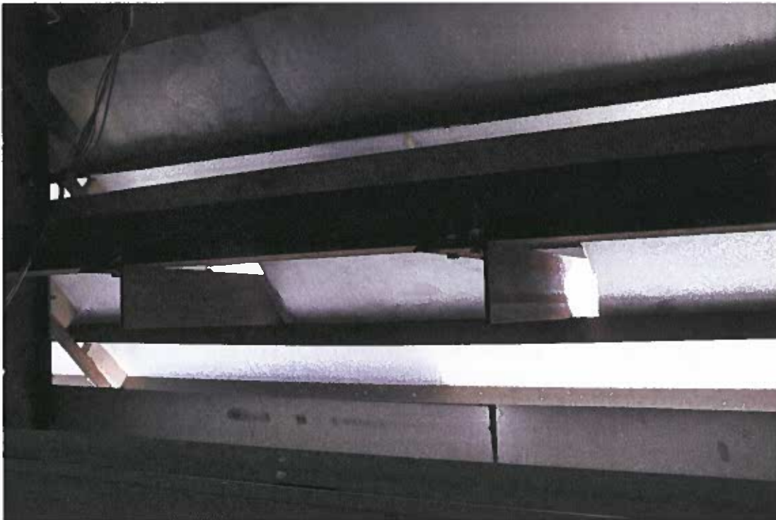
Photo 22. Detail of signage support beams and louvers, Belgian Building, 11/17/21
