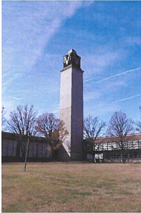
Photo 9. View of bell tower with signage, looking west, Belgian Building, 11/17/21
