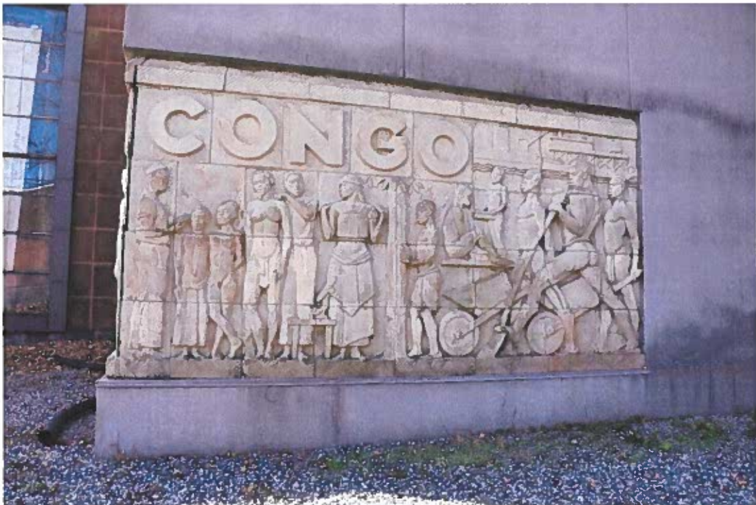
Photo 4. Detail of northeast facing panel on tower base, Belgian Building, 5/23/19
