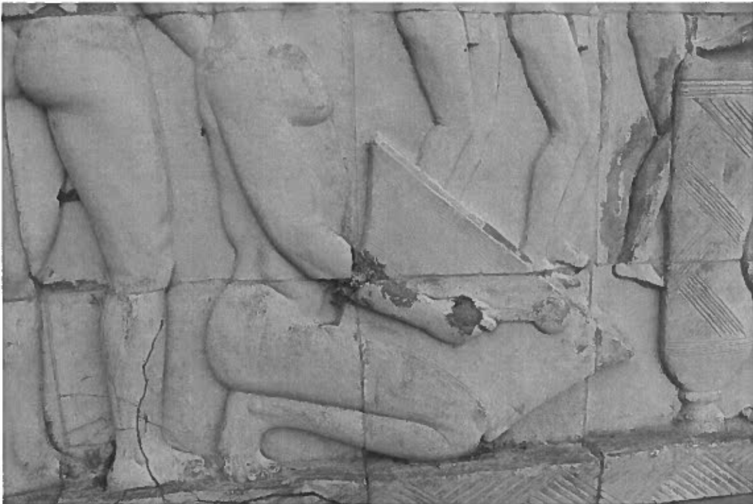
Photo 6. Detail of typical deterioration on bas-relief panel, Belgian Building, 11/17/21
