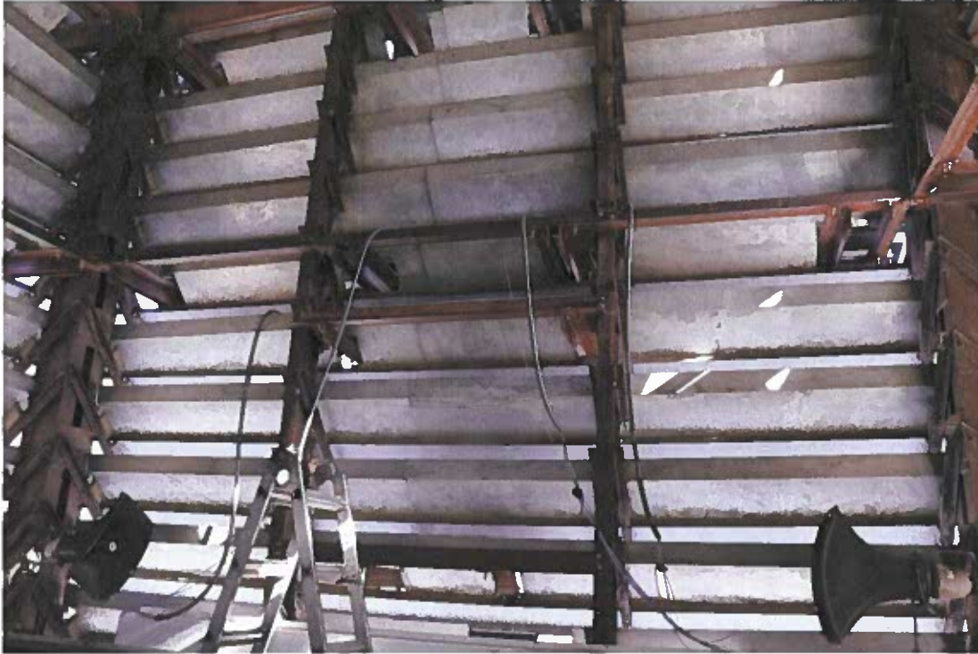
Photo 21. Detail of new signage mounts at top of bell tower, Belgian Building, 11/17/21
