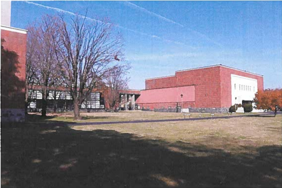
Photo 11. View of courtyard and gymnasium building, looking north, Belgian Building, 11/17/21
