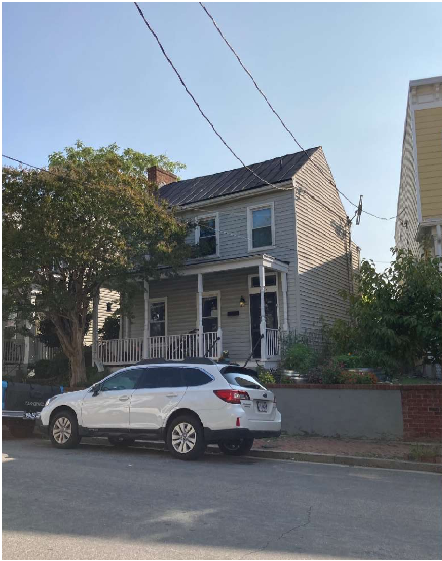
605 N 21st St. - West Elevation
