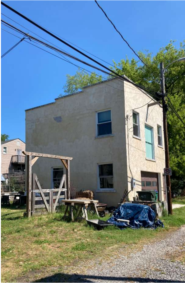
607 N 23rd St. - View from Alley
