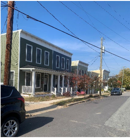
Figure 6. New construction across the street
