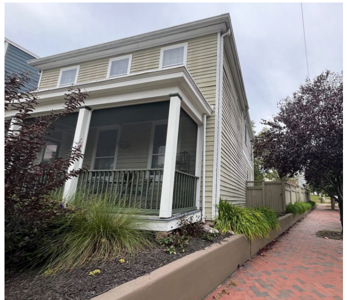
Figure 2. Front façade facing North.
