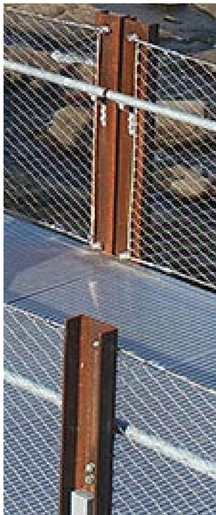
WEATHERED STEEL POSTS W/BROWN/BLACK SS NETTING AND GRAY GALV STEEL DECKING
