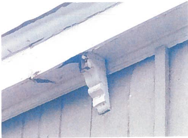
Above: Existing Bracket on the Front Facade
