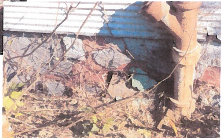
Right: Existing condition @ foundation wall
