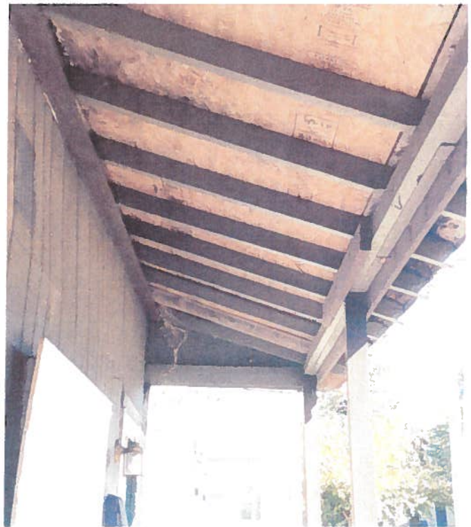
Existing condition @ Front Porch
