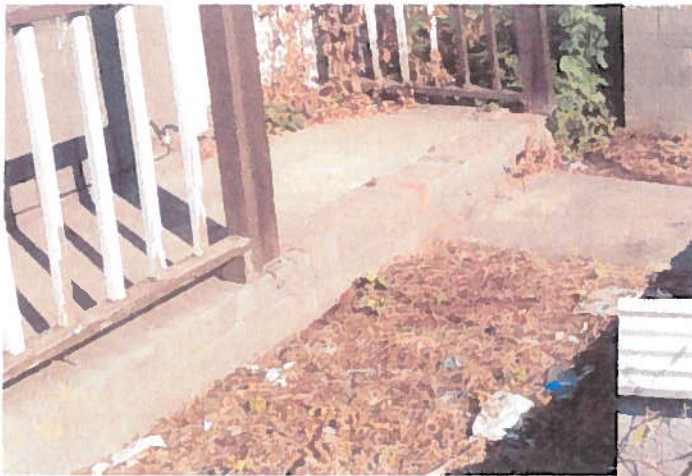
Above: Existing condition @ porch slab
