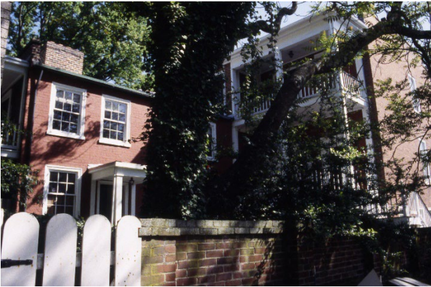
Figure 3. 2600 East Franklin Street, 1998, VCU Digital Archives. Rear Porch off former dependency present.
