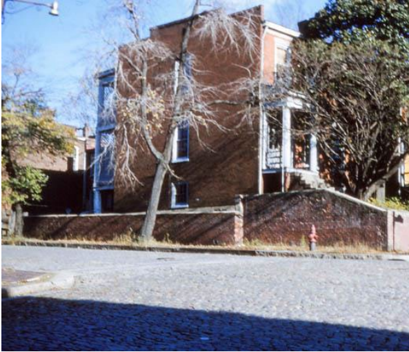
Figure 1. 2600 East Franklin Street, 1956, Valentine Museum Digital Archives. Rear porch off former dependency not present.
