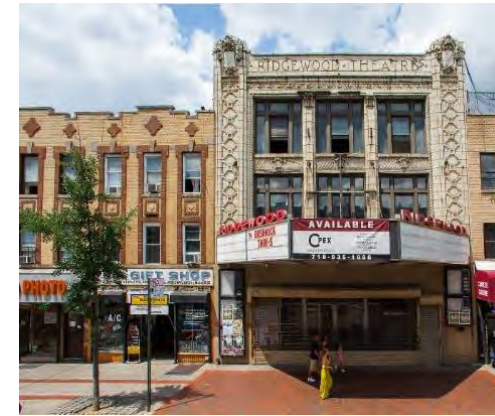
Converted Theater Apts., Queens
