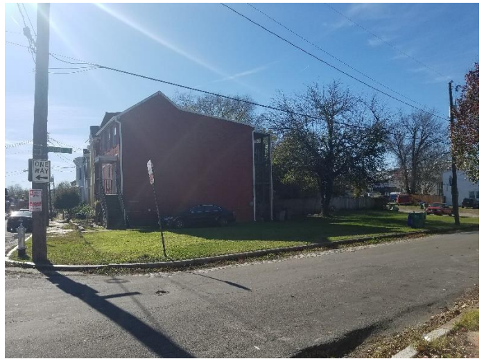
Figure 2. 618-620 North 21st Street.
