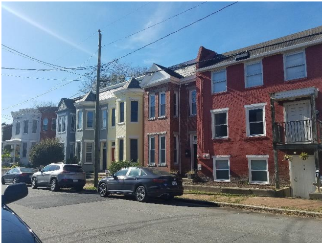
Figure 3. 608-615 North 21st Street.
