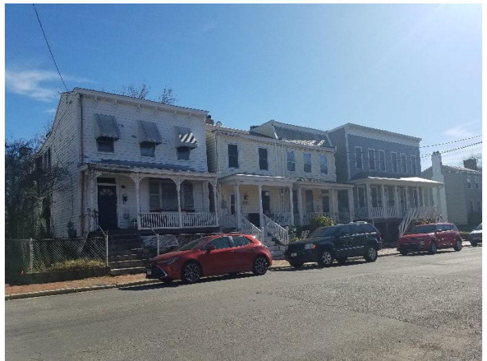
Figure 4. 611-619 North 21st Street.
