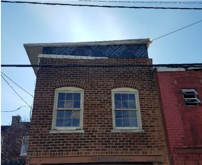
Figure 7. 2012 W. Grace St, carriage house, new cantilever.
