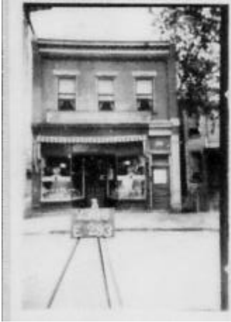
Figure 1. Assessor's photograph, ca. 1923-1956.
