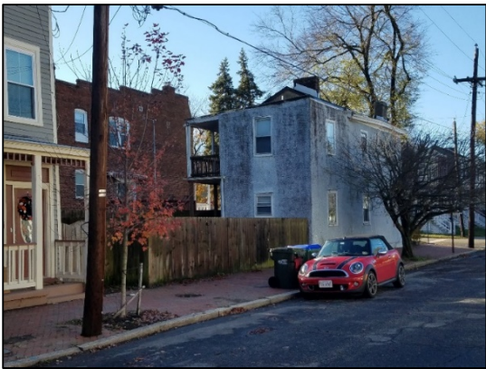
Figure 5. 2800 East Leigh Street, rear elevation, 2018.
