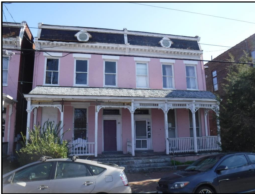
2406-2408 East Clay Street (March 2018)
