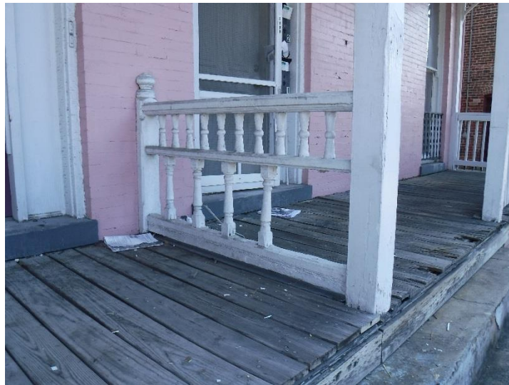
Surviving Railing at 2406-2408 E. Clay Street (March 2018)
