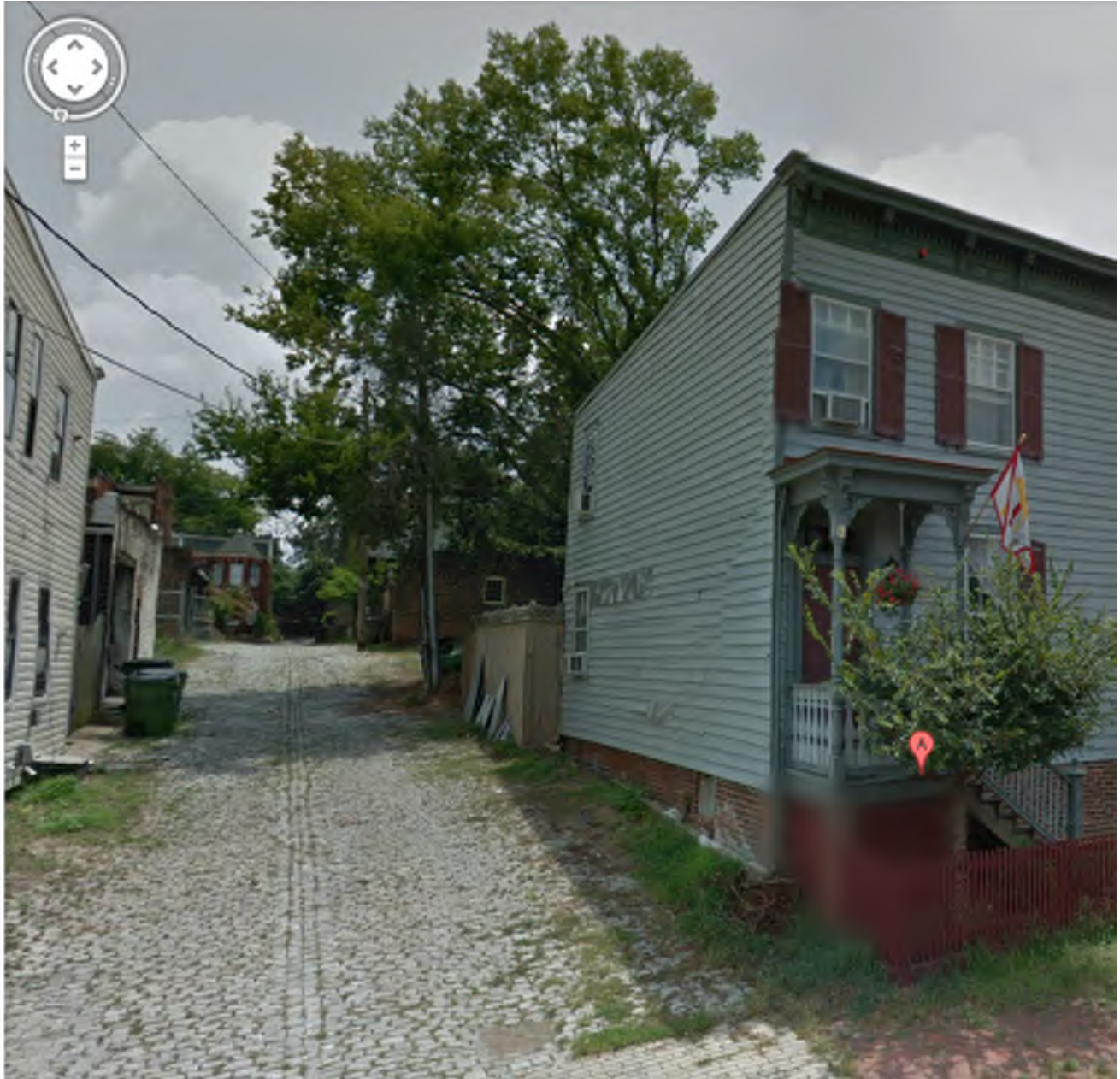
Photo of Ally Elevation – Siding and window for replacement
