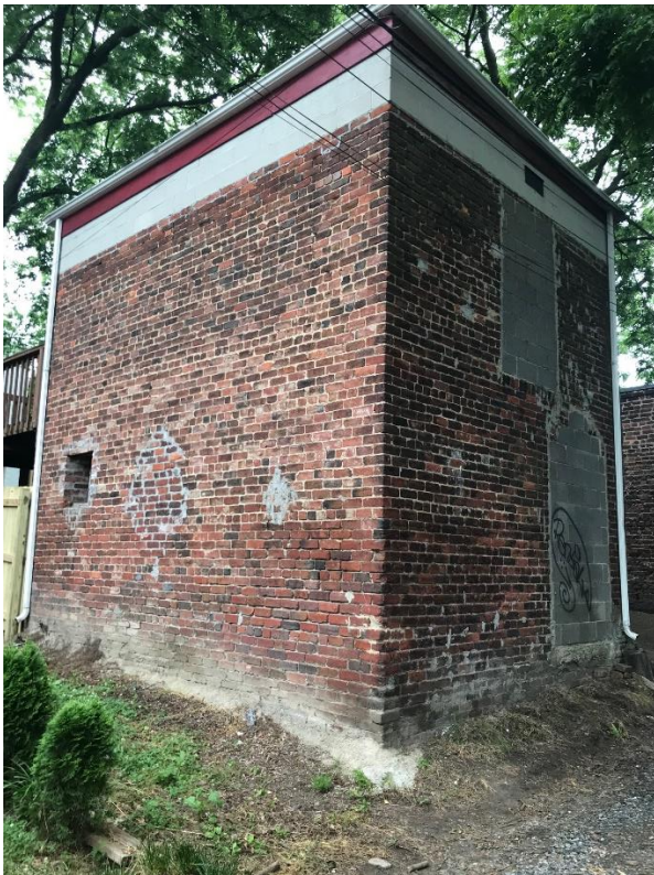
Figure 3. North and east elevations of existing carriage house
