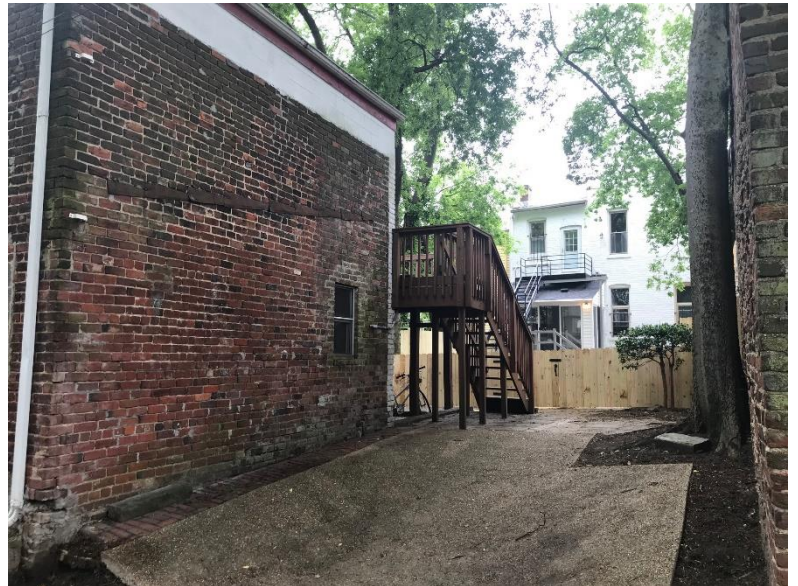
Figure 4. East elevation and deck, as viewed from alley
