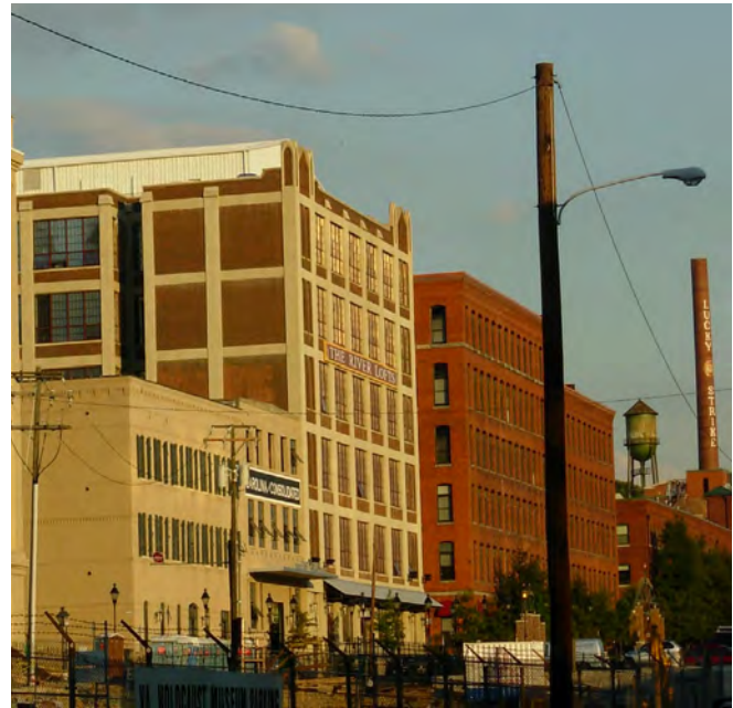
20th Century Industrial Character -- Symmetrically placed doors and windows in base, vertically and symmetrically arranged openings in the middle, and a stepped parapet at the top. Subtle variations in height, variations in color and materials to accent the organization of the elevations.
