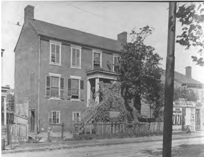
220 N. 18th Street, demolished, credit Valentine Museum
