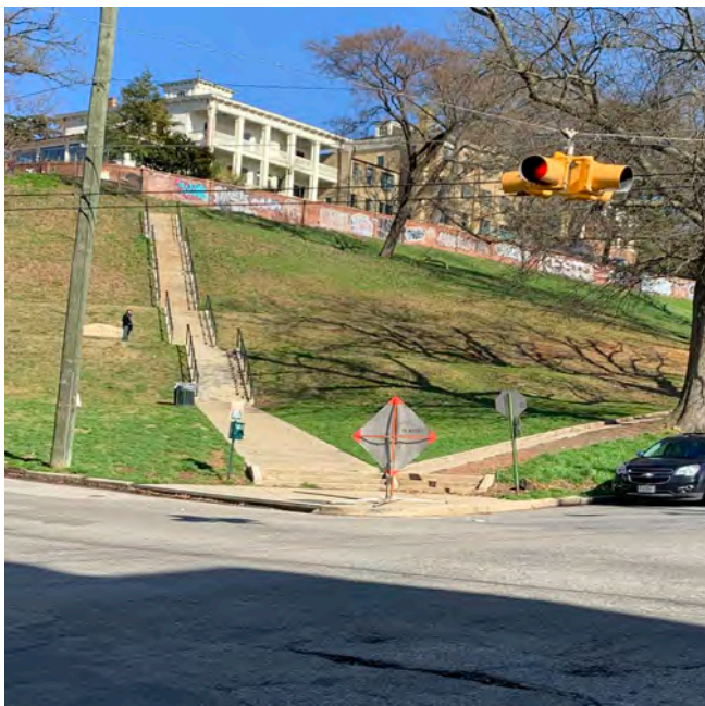
Steps from E. Franklin and N. 21st Streets to Taylor's Hill Park
