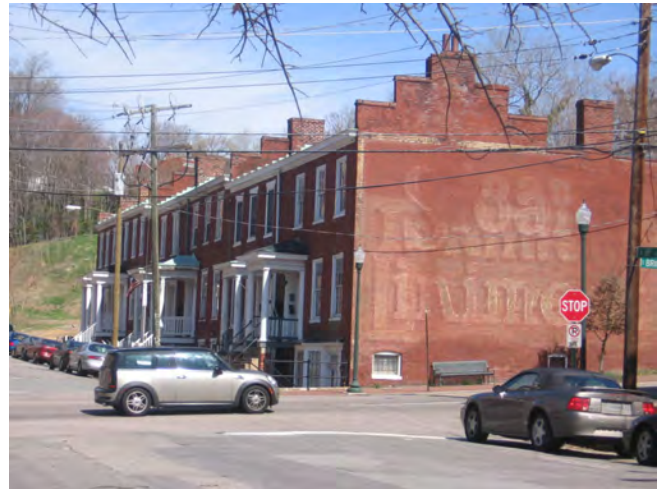
Elm Tree Row, built ca. 1853-1854 301-311 Cedar Street
