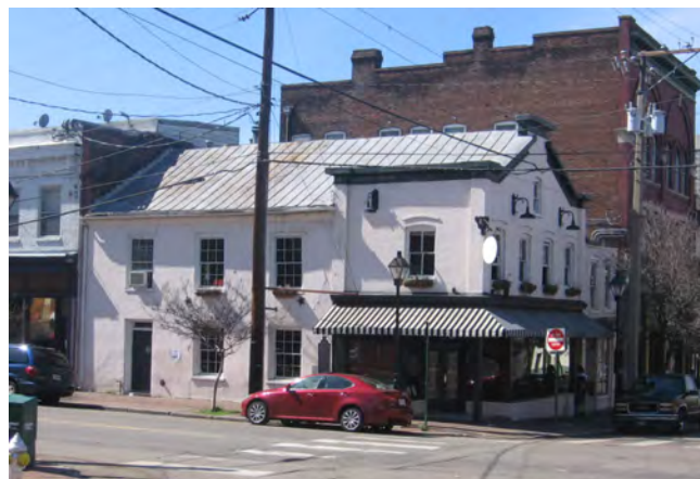
Whitlock’s Factory, built ca. 1817 1719 E. Franklin Street
