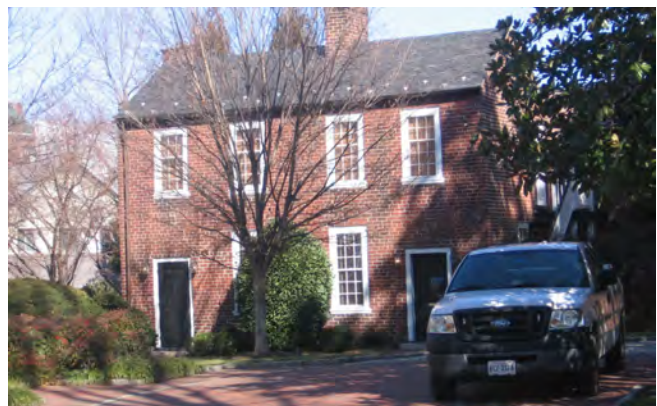
Kitchen and Quarters, Adam Craig House, built ca. 1815
