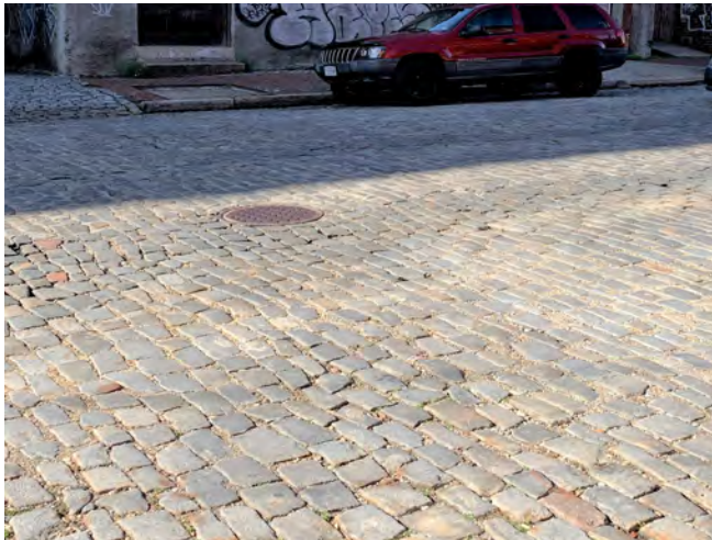
Restored cobblestone street
