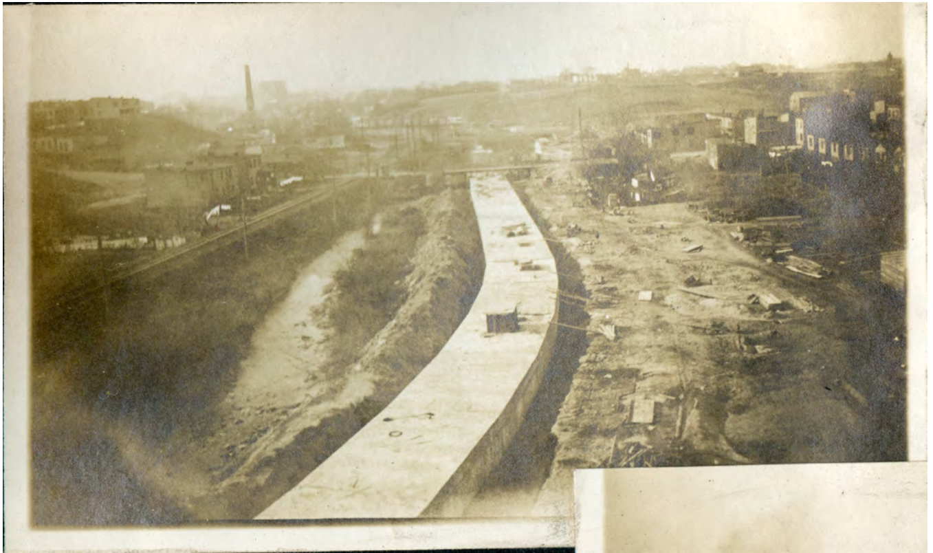
Channelizing Shockoe Creek in the 1920s, credit Valentine Museum
