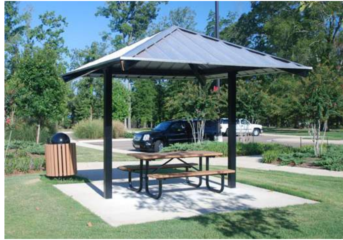
SMALLER PICNIC SHELTER (12. FT. x 12 FT. ) GABLE ROOF SUNSHELTER BY POLIGON. WILL HAVE TWO PICNIC TABLES EACH.
