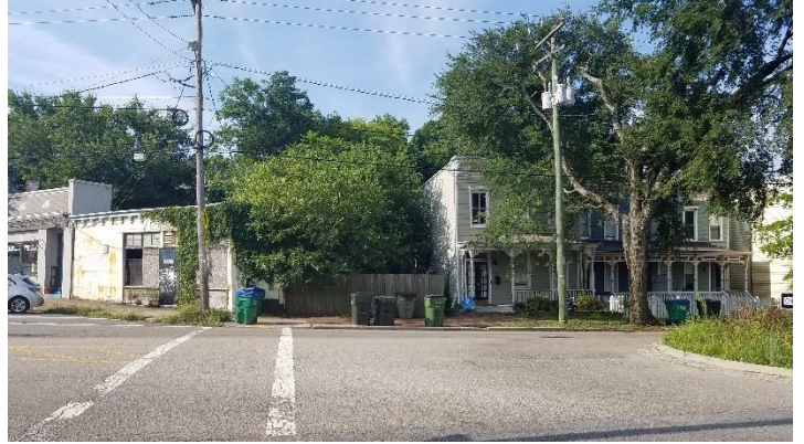
Figure 2. 2211 and 2203-2205, 2207, and 2211 Jefferson Street.
