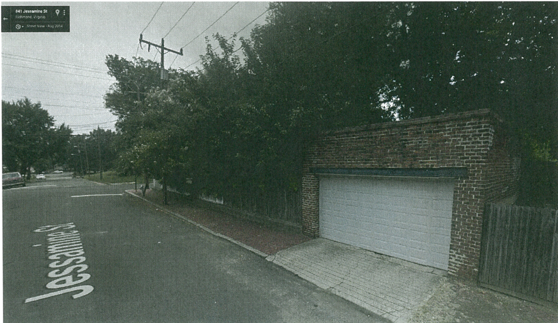
BRICK SHED WITH OPERABLE GARAGE DOOR
