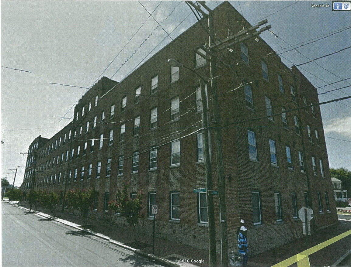
FOUR STORY BUILDING
