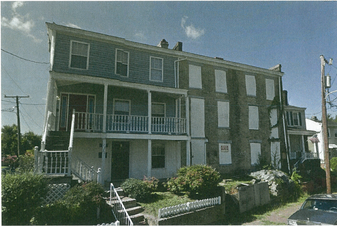
COVERED, SECOND STORY PORCHES
