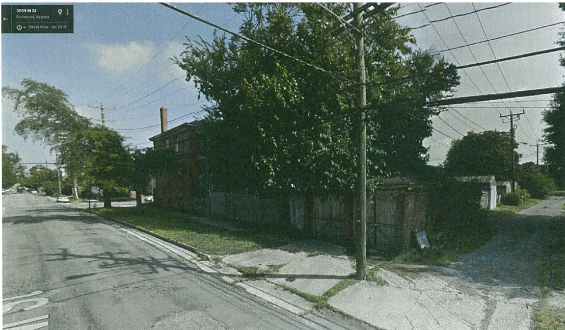
BRICK SHED WITH OPERABLE WOOD DOORS
