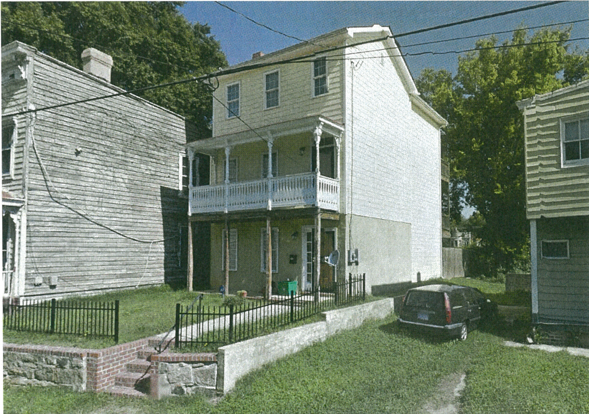
COVERED, SECOND STORY PORCHES
