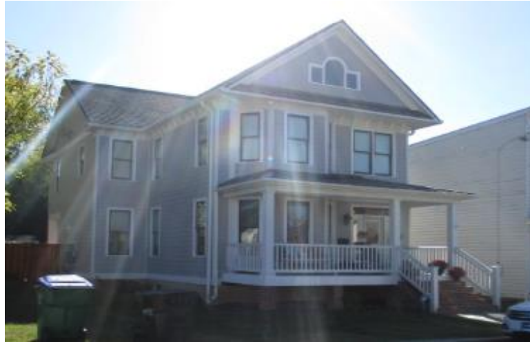
Figure 3: CAR approved dwelling at 2317 Carrington Street
