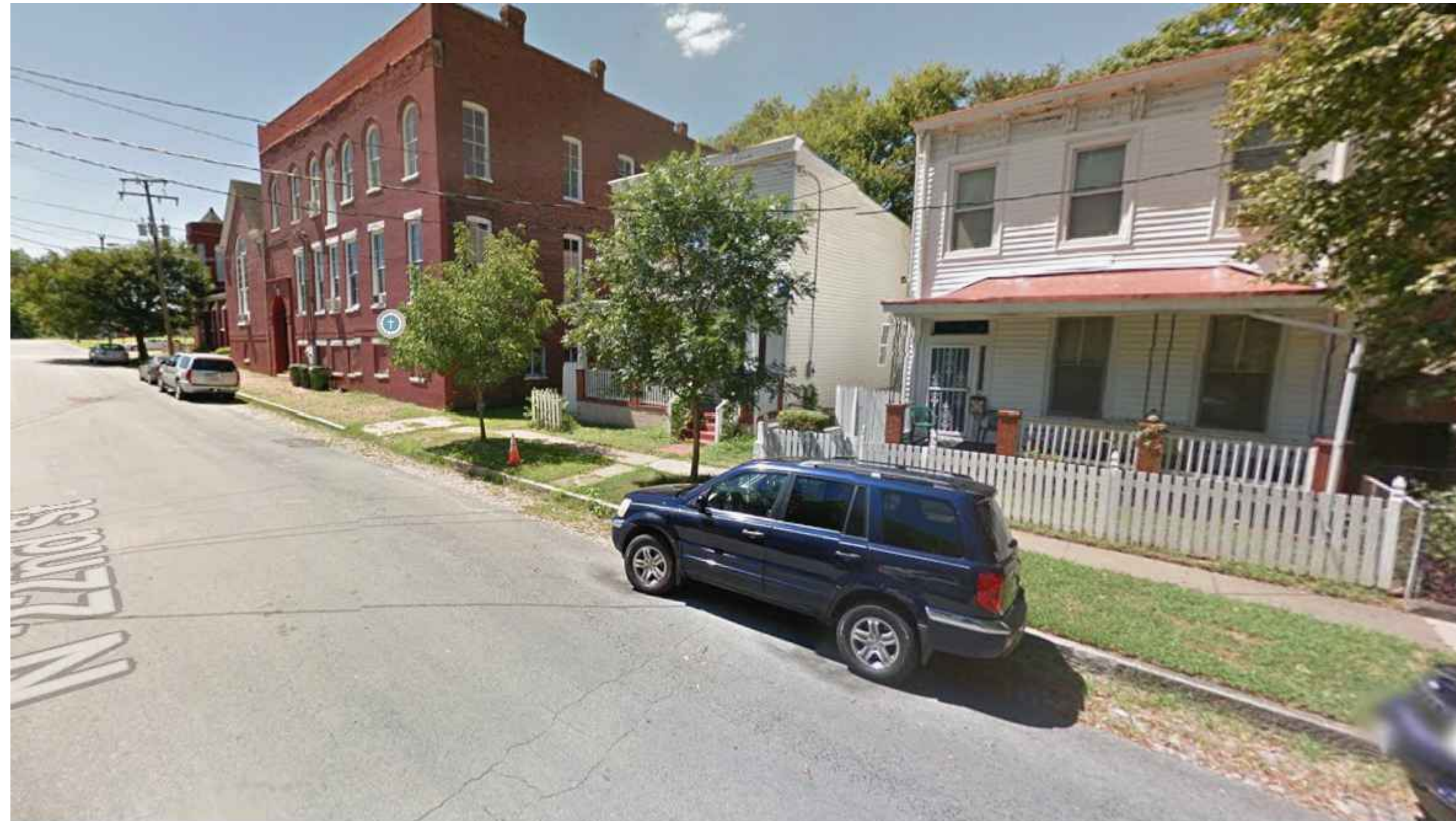
ADJACENT PROPERTIES AND STREETScape
