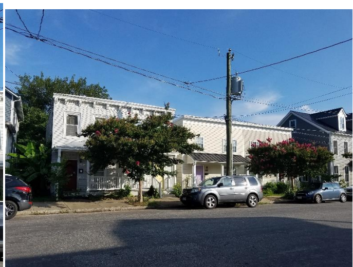
Figure 6. 620-622 North 29th Street.
