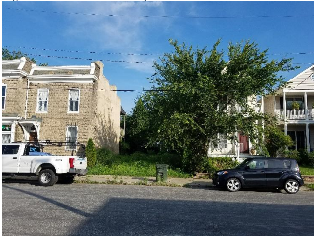
Figure 3. 606-608 North 29th Street.
