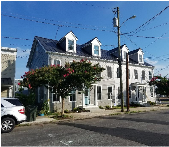
Figure 7. 634-638 North 29th Street.
