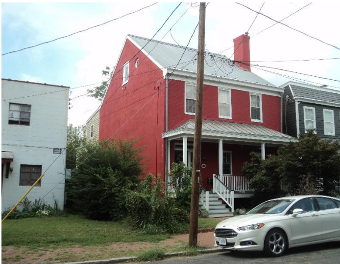
Figure 9. 510 North 29th Street.
