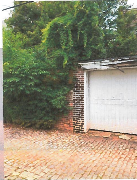
View of 1821 Monument from alley looking west
