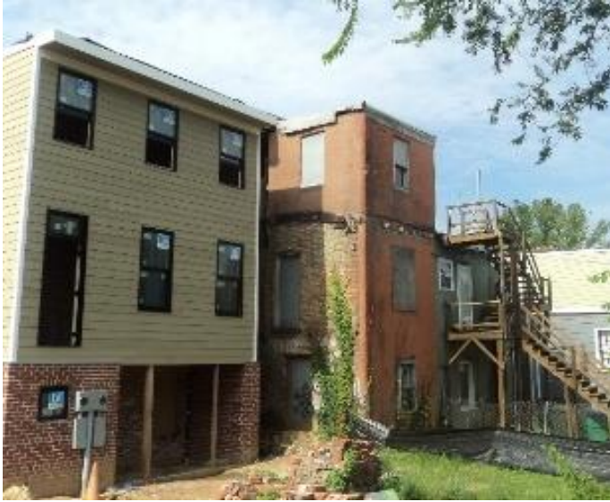
Figure 5. Rear elevation, viewed from Pink Street
