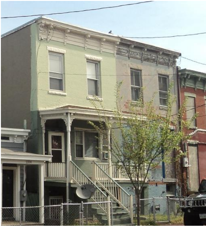
Figure 3. Porch at 2316 Venable Street
