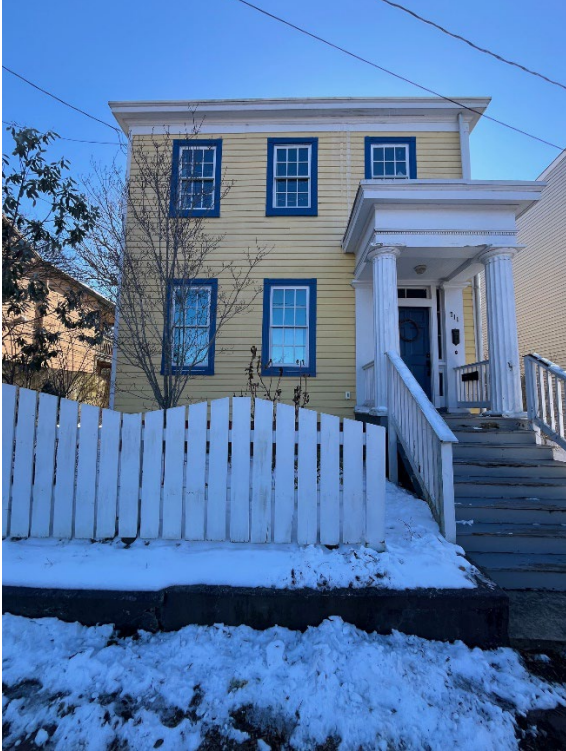
Figure 1. 711 North 26 th Street Façade, February 2025.
