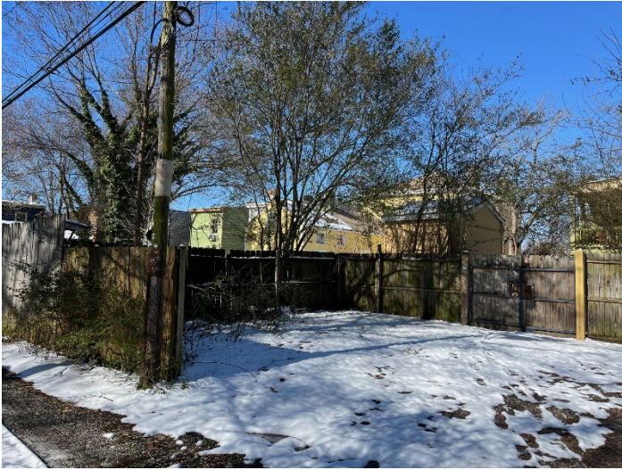
Figure 3. View of existing rear addition from the rear alley.
