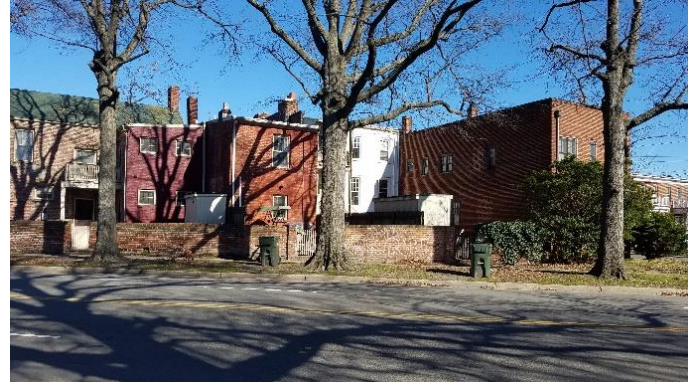
Figure 8. Rear of buildings at 101-105 West Jackson Street, view across Chamberlayne Parkway.
