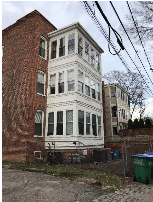
Figure 4. 2011 Monument Ave, enclosed rear porch.
