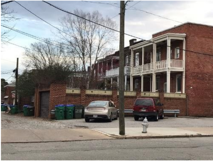
Figure 5. 2000 Block Monument Avenue, even side, rear elevations.
