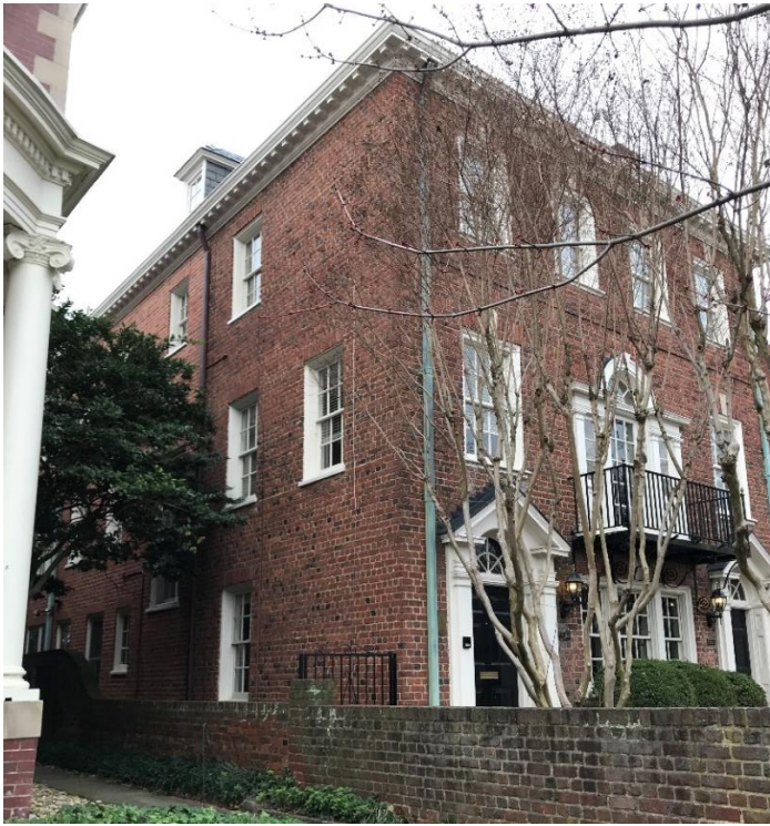
Figure 1. Façade and east elevation.
